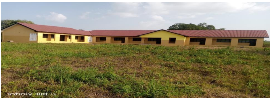
Construction of 1No. 6 Unit Classroom Block with Ancillary at Quaterpe
