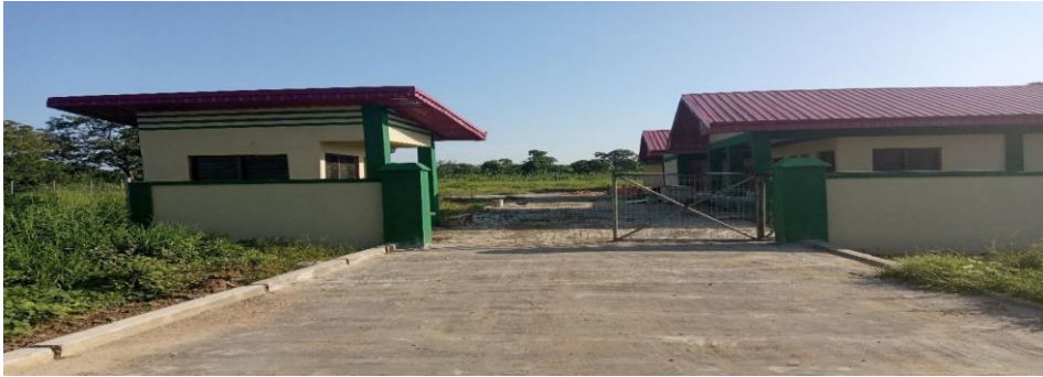
CONSTRUCTION OF CASSAVA PROCESSING FACTORY UNDER
