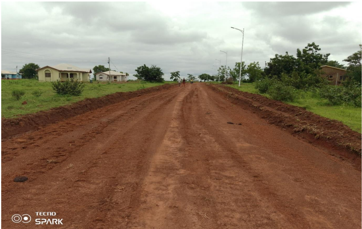
Re-shaping of Karaga Girls Model School Junction to the school and others (3.00km)
