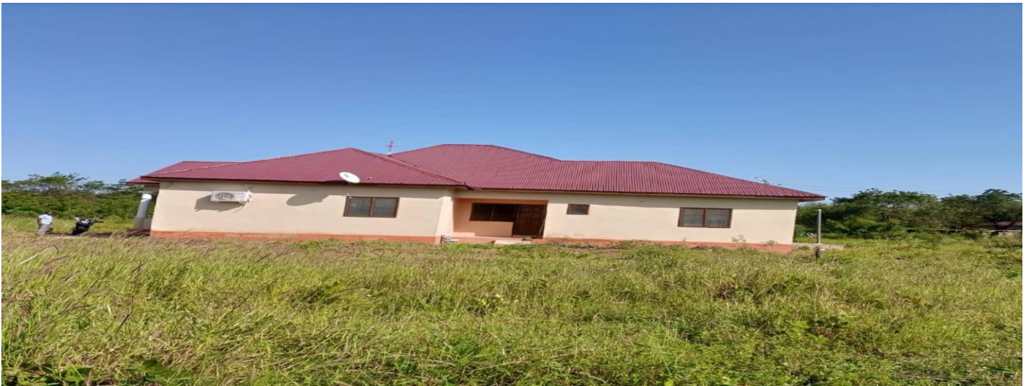
Completed and Furnished Doctor Bungalow at Gambaga
