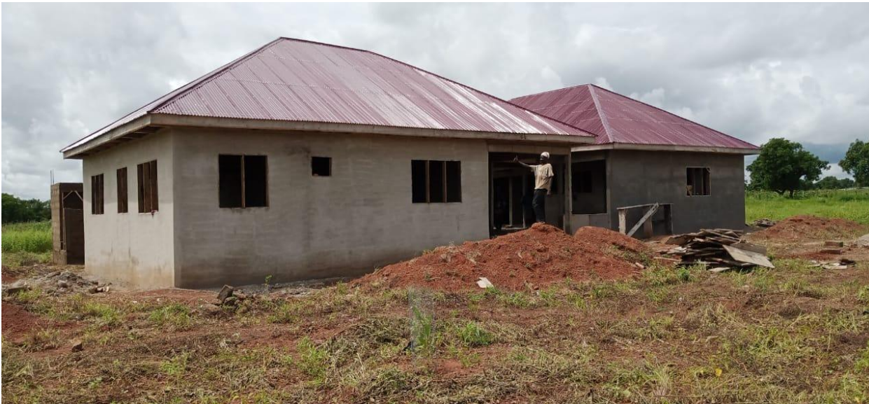
Construction and furnishing of CHPS Compound at Boku (70% Completed)
