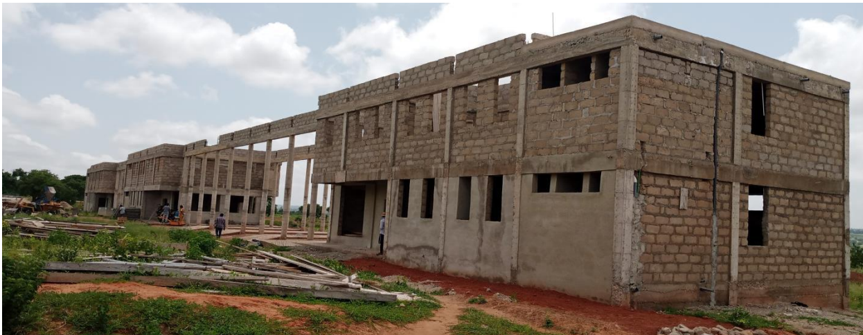
Construction of Bus Terminal, Public Washrooms and Paving at Naalerigu (46%)
