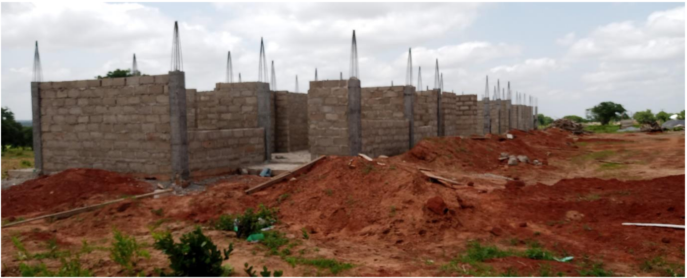
Construction of 2-storey Commercial Building, drain and Paving Works at Nalerigu (20%)
