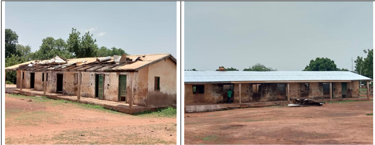
Re-roofed storm damaged 1 no. 3unit classroom block at Kpariritinga Primary School
