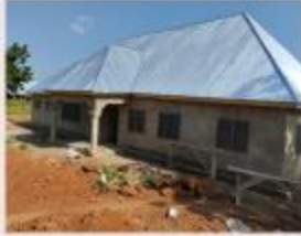
DISTRICT HEALTH ADMINISTRATION BLOCK CONSTRUCTED AT BUNKPURUGU
