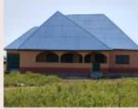
DISTRICT FINANCE OFFICER'S BUNGALOW REHABILITATED
