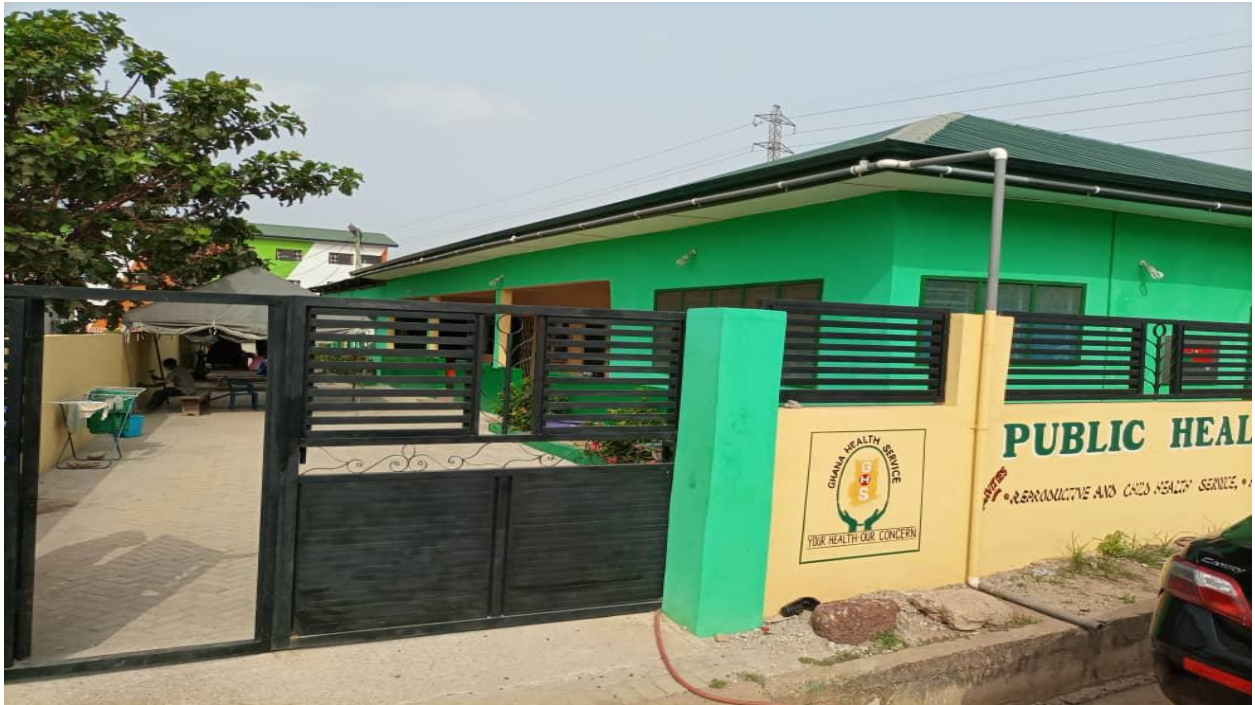
Figure 1.6 Renovated Mallam demonstration clinic.
