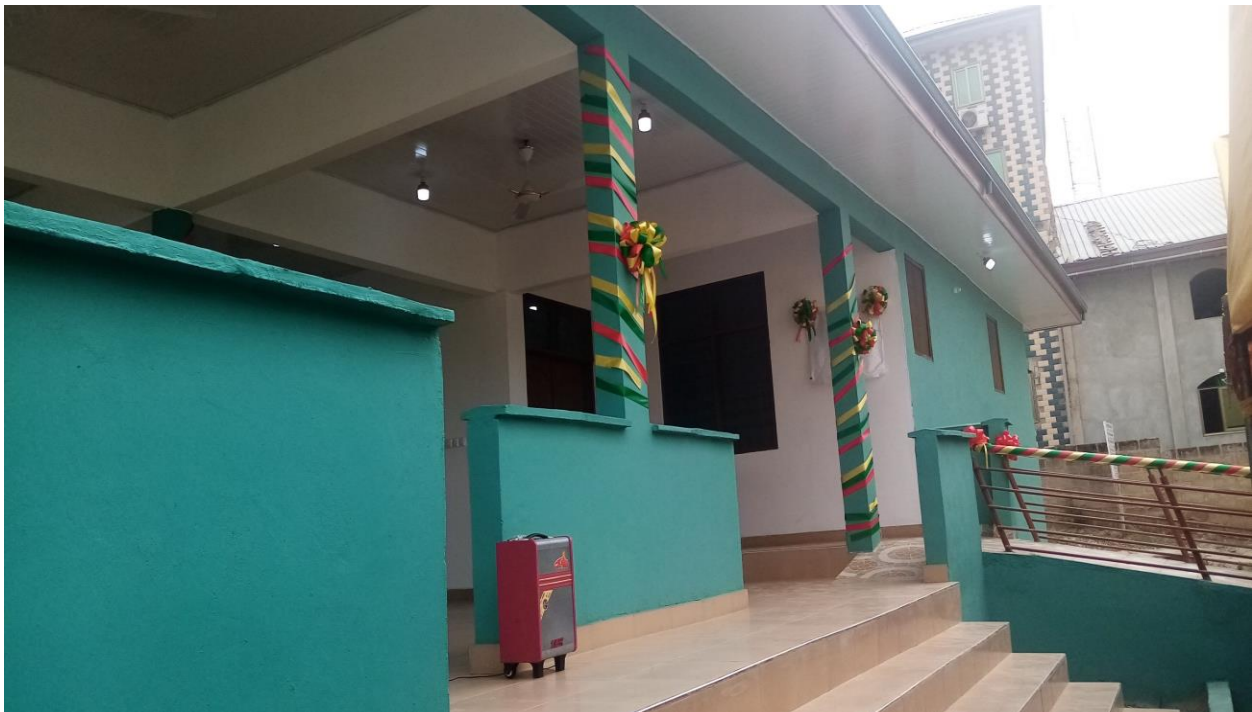
Figure 1.3 Completed 6No. Bed Capacity maternity ward, OPD Pavilion at Oblogo Clinic.
