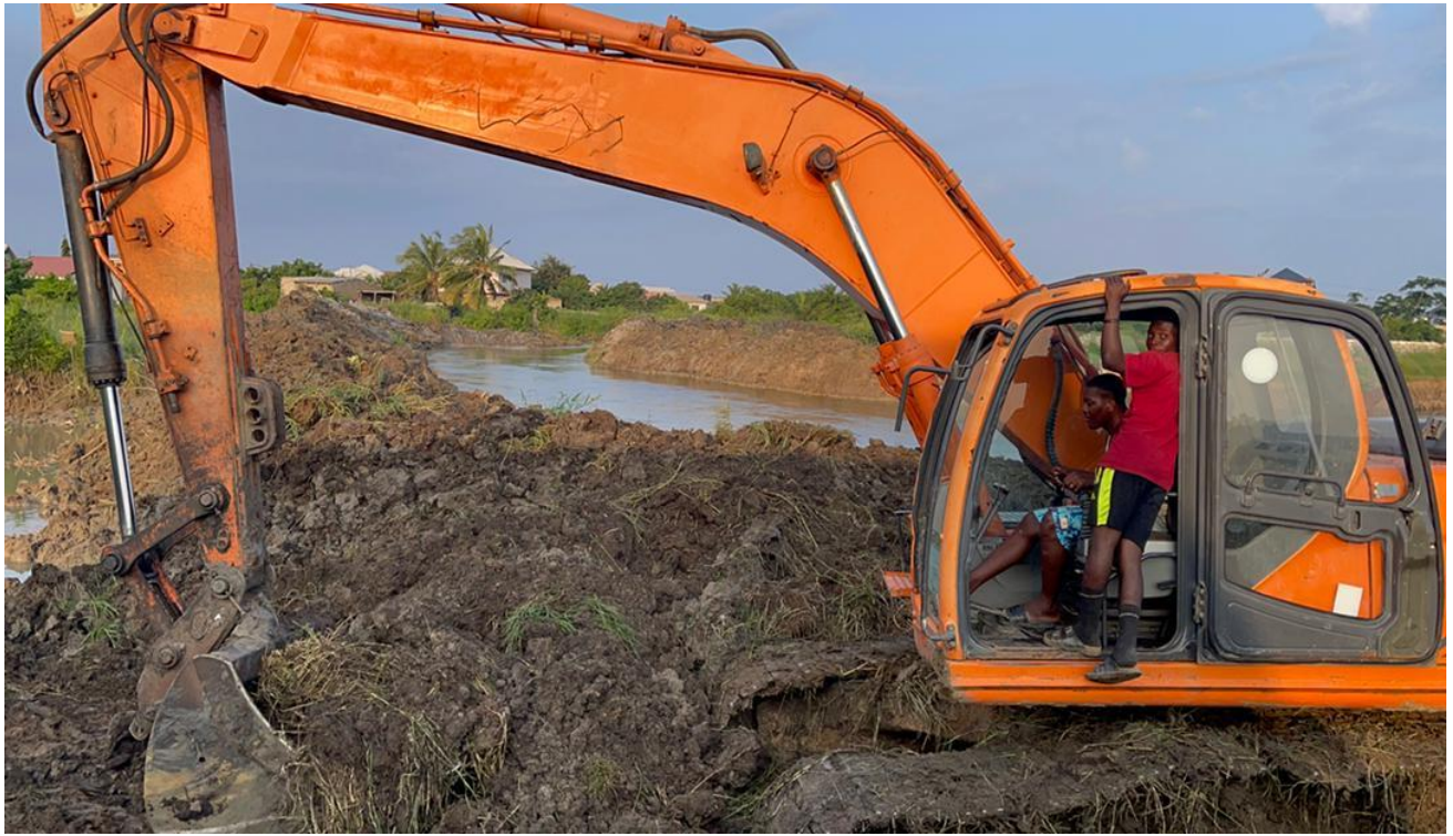
Figure 1.10 Dredged 1km earth channel drain at Tetegu
