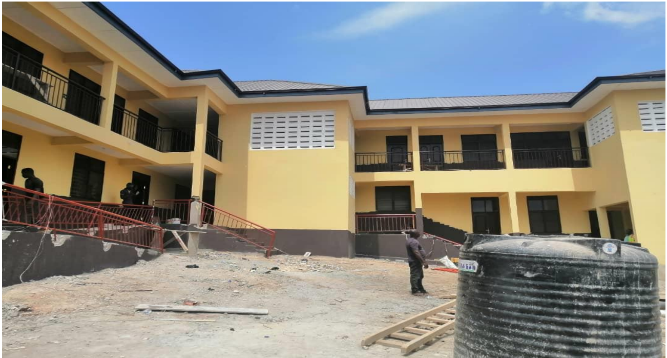
Figure 1.2 Completed 2- Storey 11-Unit Classroom block at Gonse for quality education
