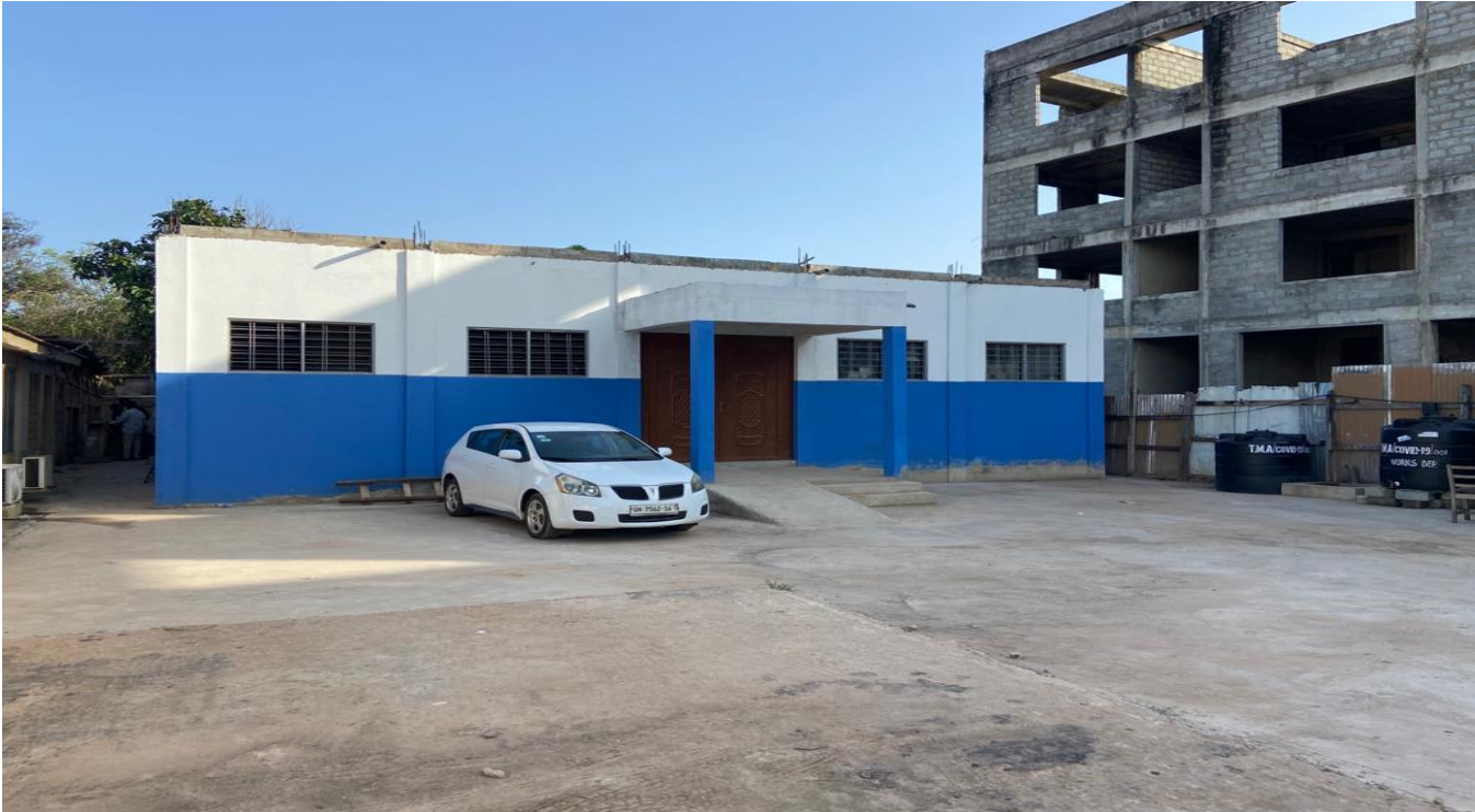
Constructed 1 No. 2 storey office stores with ancillary facilities
