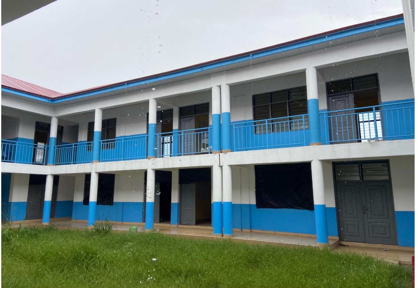
Constructed 1 No.6 Unit Kg Classroom Block at Tema Manhean Presby
