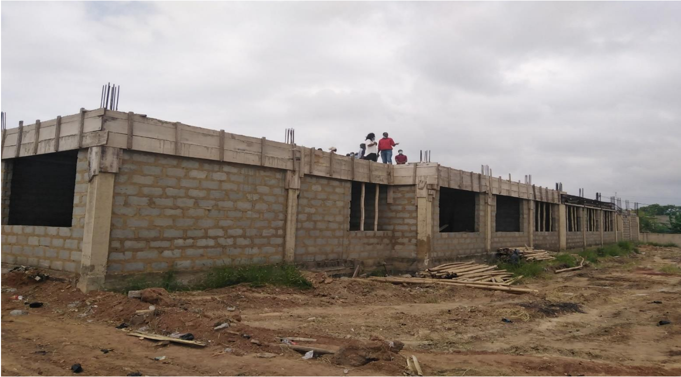
Constructed 1No. 2 storey 12 unit classroom block at Community 7, No.1 & 2 JHS
