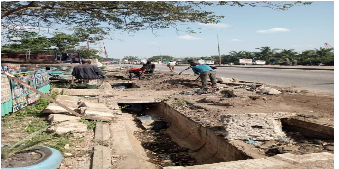
Rehabilitated damaged sewer system
