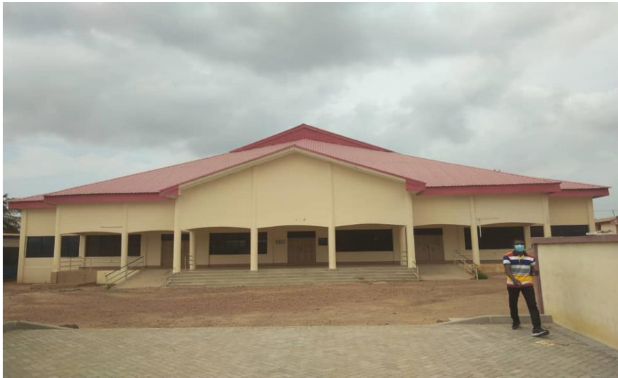
REHABILITATED TETTEH OCLOO SCHOOL FOR THE DEAF DINING HALL AT ADJEI-KOJO (DACF)
