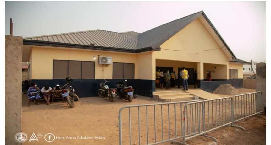
CONSTRUCTED A POLICE STATION AT ADJEI KOJO (IGF)
