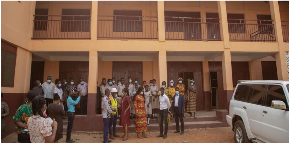
CONSTRUCTED 2 STOREY 12 UNIT CLASSROOM BLOCK AT ADJEI KOJO
