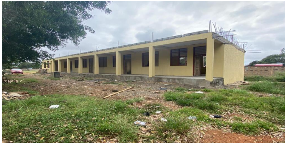
SECTIONAL COMPLETION OF 3-UNIT CLASSROOM BLOCK AT STAR SCHOOL, COMM.5
