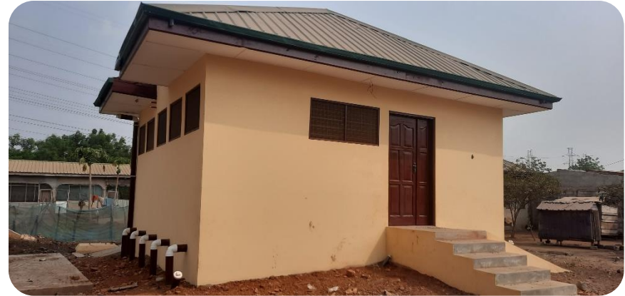
Constructed 10 Seater Water Closet Facility at Doryumu
