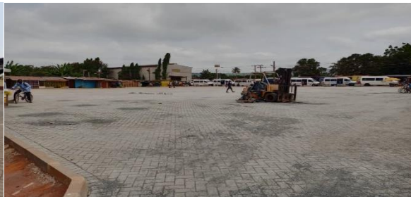
CONSTRUCTED RIGID PAVEMENT AT ABOKOBI LORRY PARK
