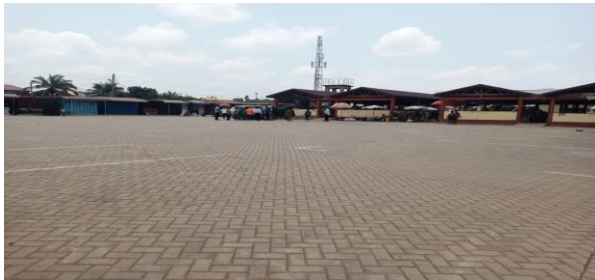
CONSTRUCTED RIGID PAVEMENT AT TAIFA LORRY PARK
