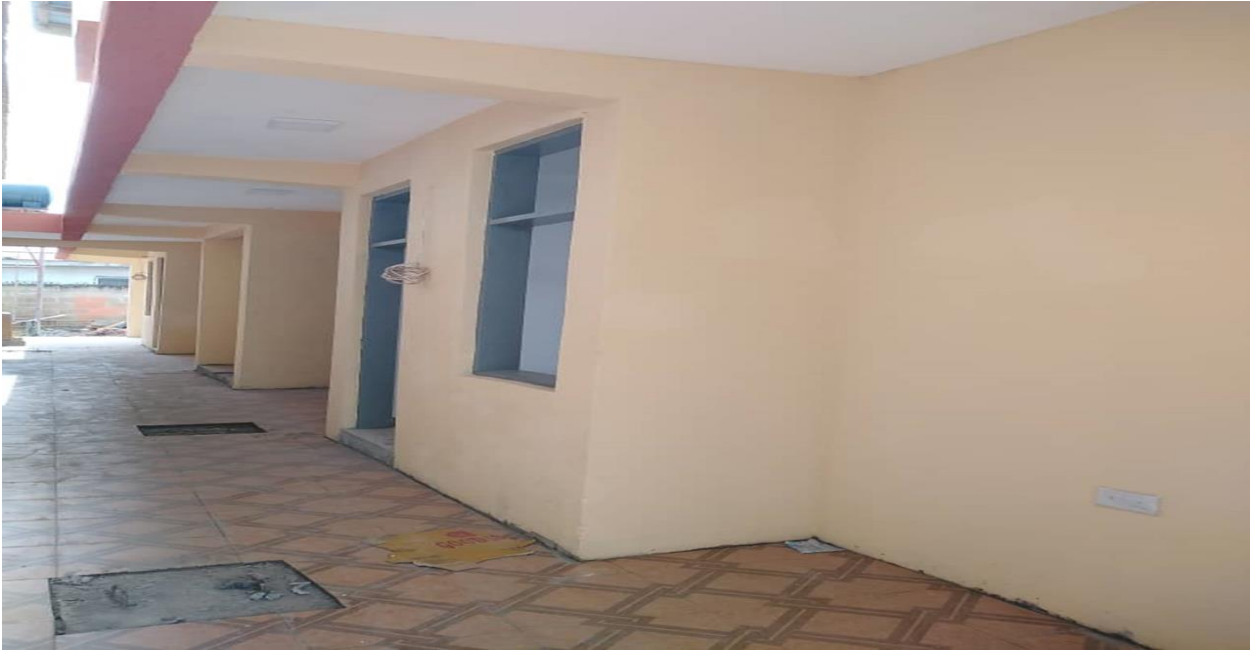
Picture 2: Constructed 4-Unit Holding Centre at Kwashiebu
