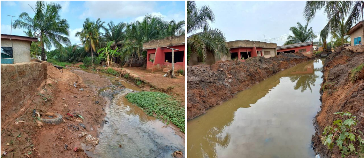
Picture 5: Dredging of water course at Auntie Aku
