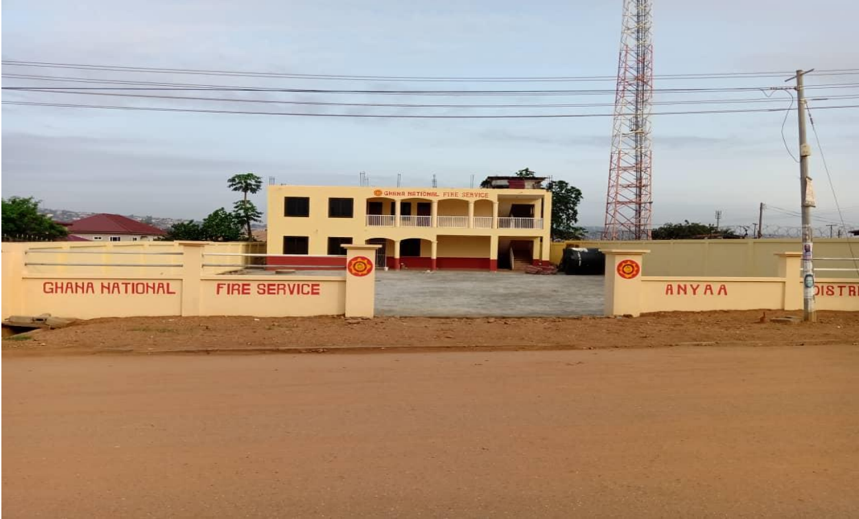
Picture 3: Constructed 2-Storey Fire Service Station at Anyaa
