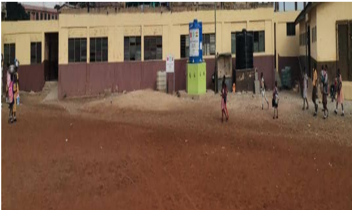
CONSTRUCTED OF 6 UNIT CLASSROOM BLOCK – MODEL SCHOOL
