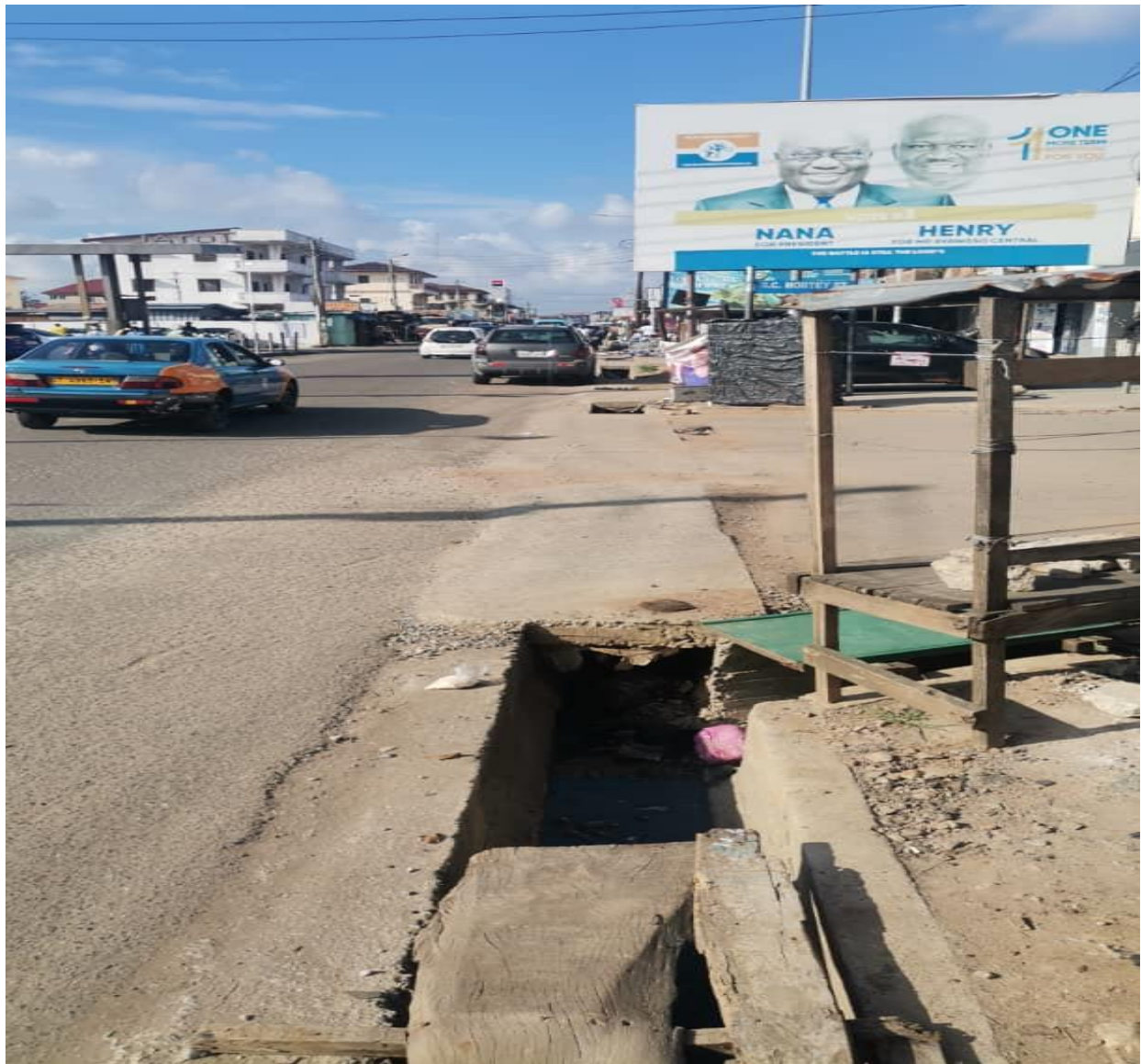
Constructed 0.45KM, 0.6 concrete U-Drain at Newtown
