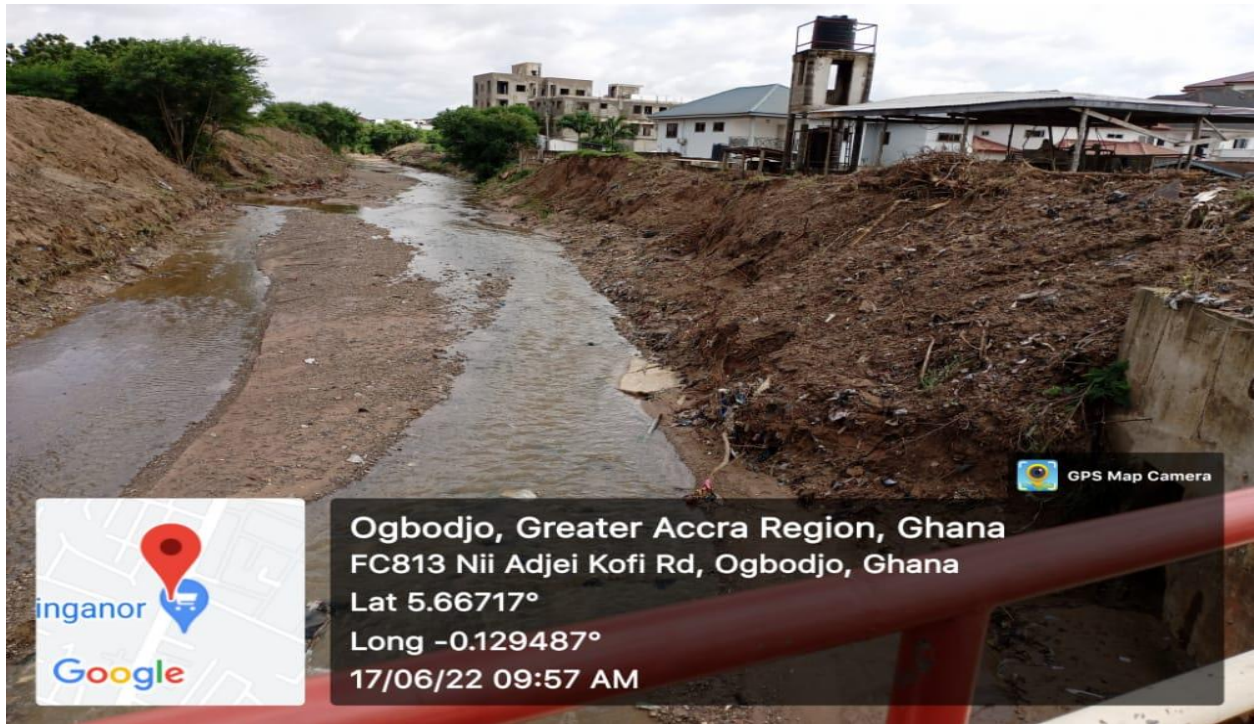
DREDGED WORKS AT OGBOJO
