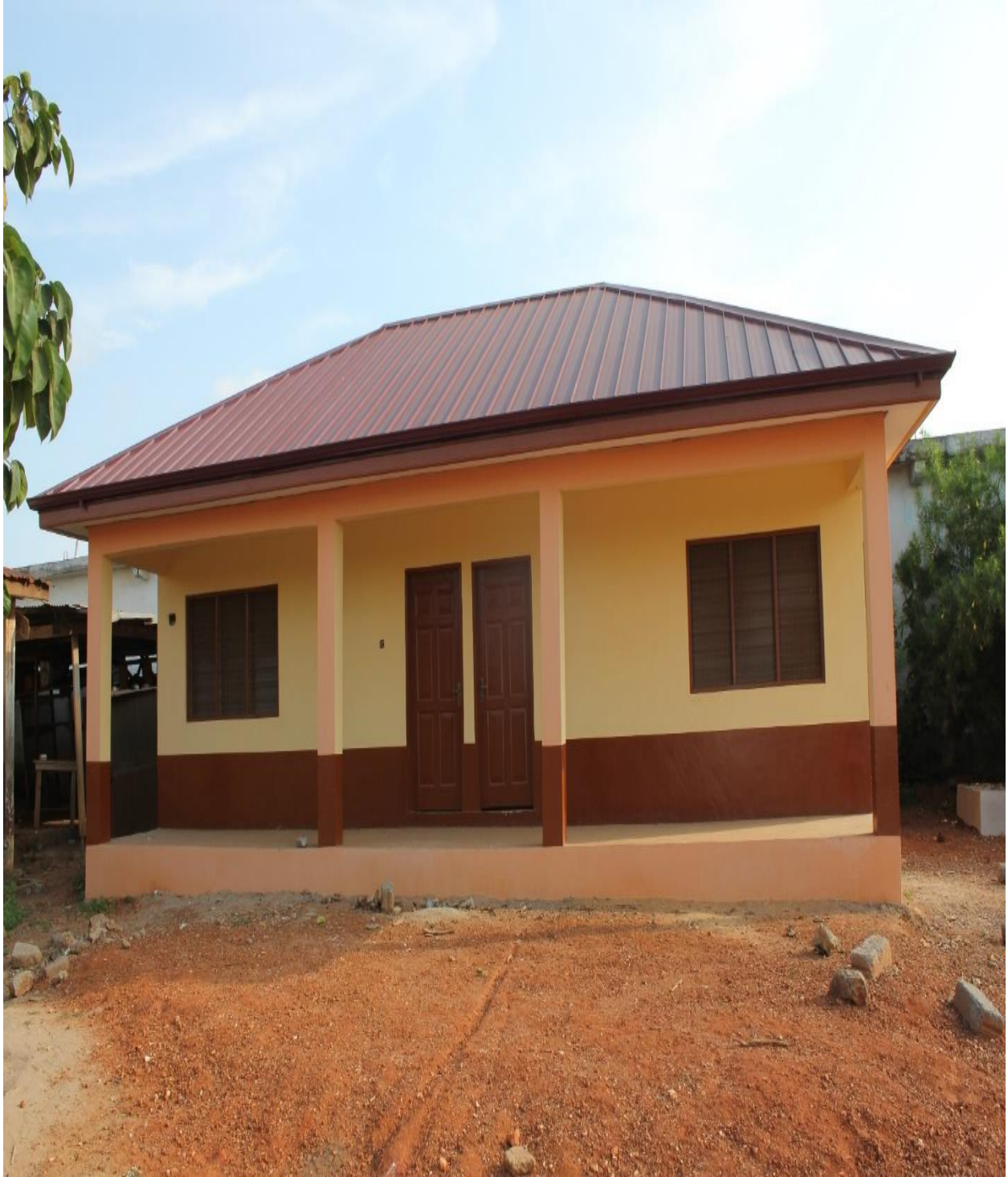
CONSTRUCTED 1NO. 2-UNIT KITCHEN (UNDER SCHOOL FEEDING PROGRAMME) AT ICODEHS SCHOOL IN ADENTAN
