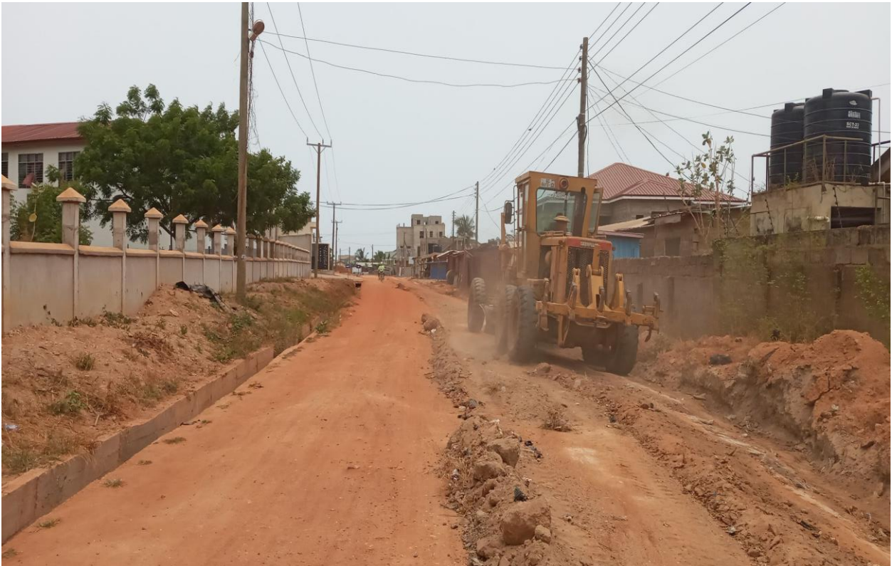
GRADED OF SOME SELECTED ROADS- LAKESIDE NEW NATION, FAIR HAVEN ESTATES AREA
