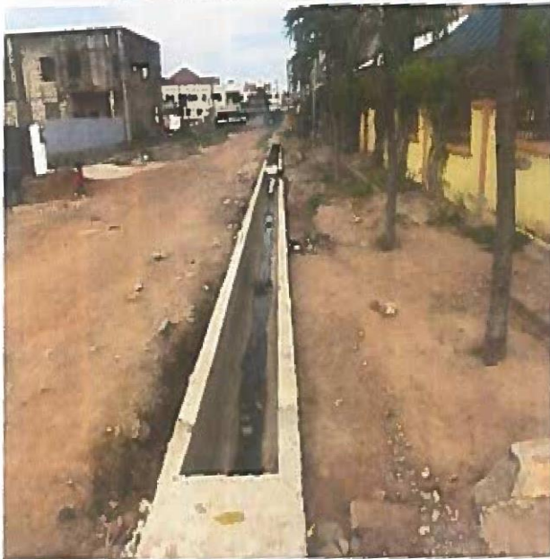
CONSTRUCTED 0.6 U-DRAIN BEHIND OGBOJO POLY CLINIC THROUGH THE COMMUNITY
