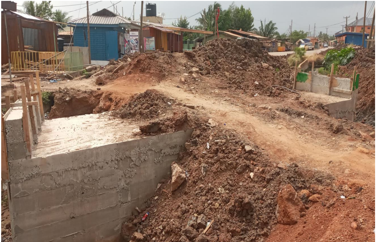
CONSTRUCTED CULVERT AT ACCOUNTANCY DOWN
