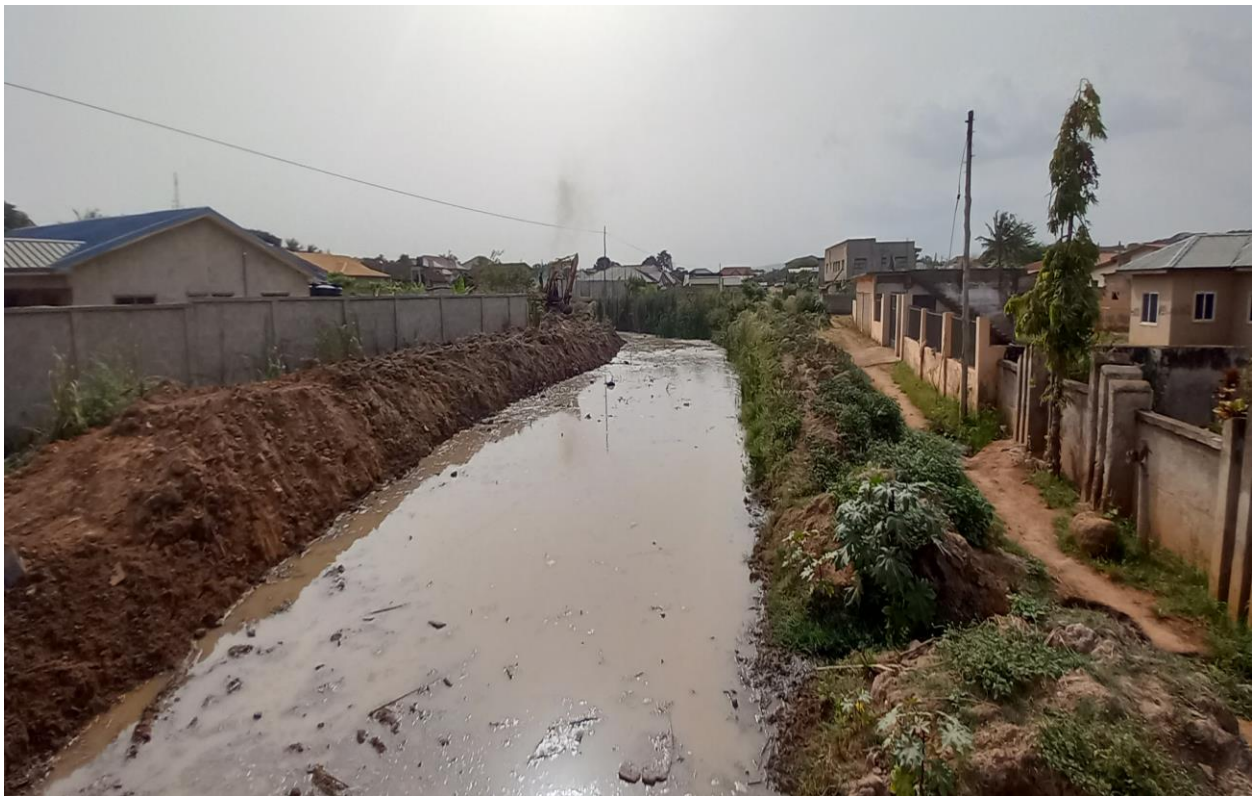
DREDGED WORKS AT FRAFRAHA PRISON JUNCTION
