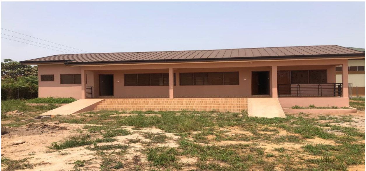
CONSTRUCTED FISH DEMONSTRATION CENTRE AND ADMINISTRATION BLOCK AT AMRAHIA (PHASE 1 &2)
