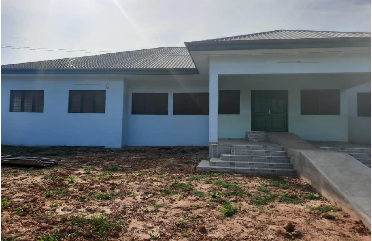
MATERNITY WARD AT FAFRAHA COMPLETED AND IN USE
