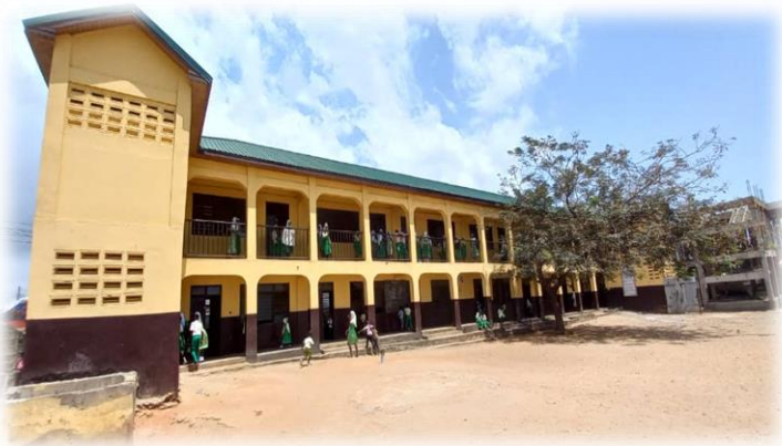
COMPLETED THE CONSTRUCTION OF 1 STOREY CLASSROOM BLOCK FOR AL-RIYAHD SCHOOL
