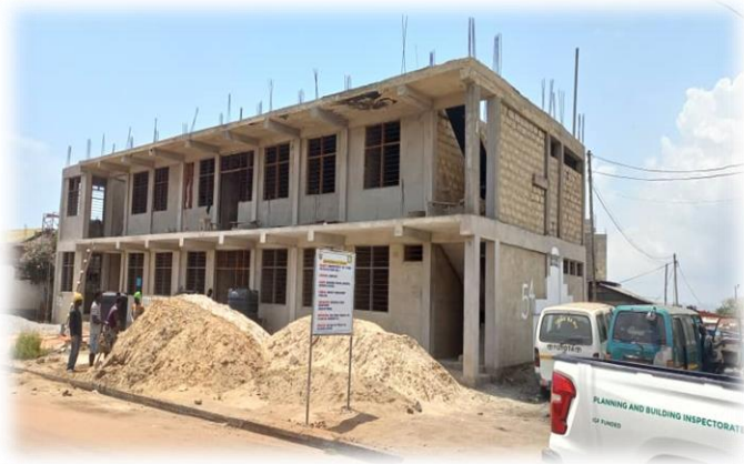
CONSTRUCTION OF 2 STOREY POLYCLINIC AT MAMBROUK (PHASE 1 COMPLETED)
