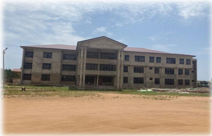
CONSTRUCTION OF OFFICE BUILDING COMPLEX (80% COMPLETED)
