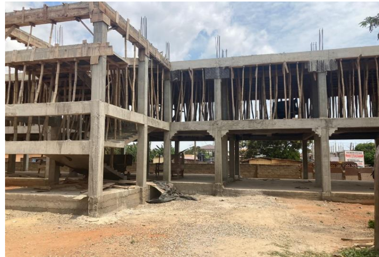
CONSTRUCTION OF 2 STOREY CLASSROOM BLOCK AT AL-RIYAAD BASIC SCHOOL (PHASE I COMPLETED)
