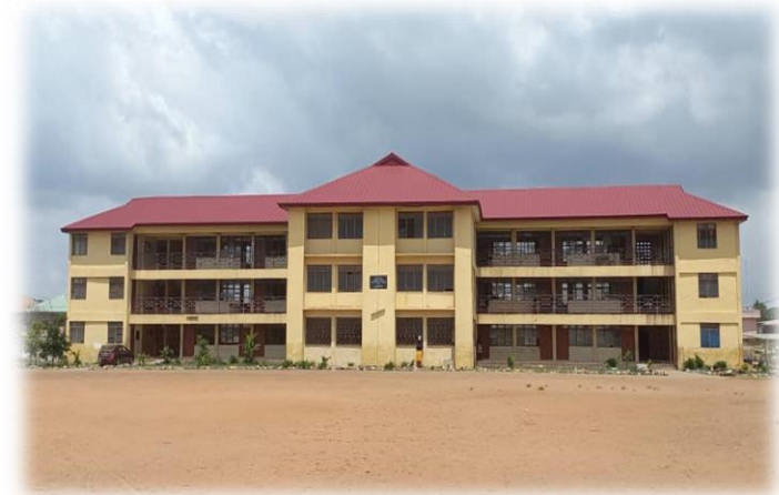
REROOFED 2 STOREY CLASSROOM BLOCK AT SALVATION SCHOOL (BARACK OBAMA SCHOOL)
