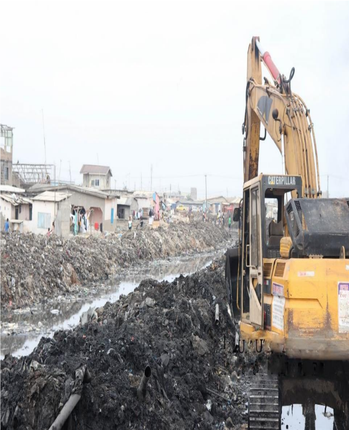
De-silting and dredging of storm drains within the municipality – 100% completed
