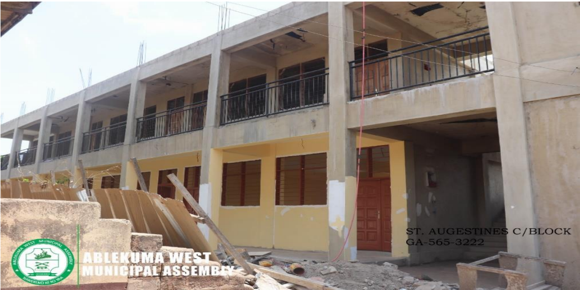
Construction of 1No. 2-Storey 6-Unit Classroom Block @ St. Augustine Ang. – 92% Completed
