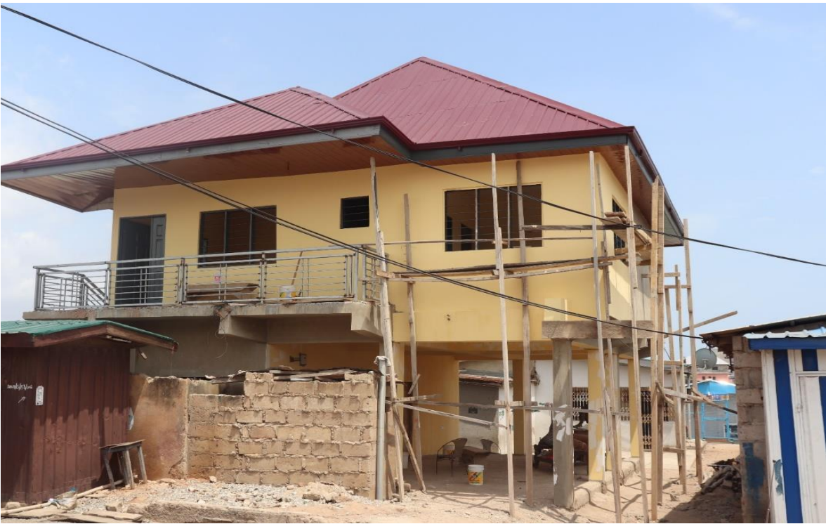
Completion of Community Centre at Nasarawa – 95% completed
