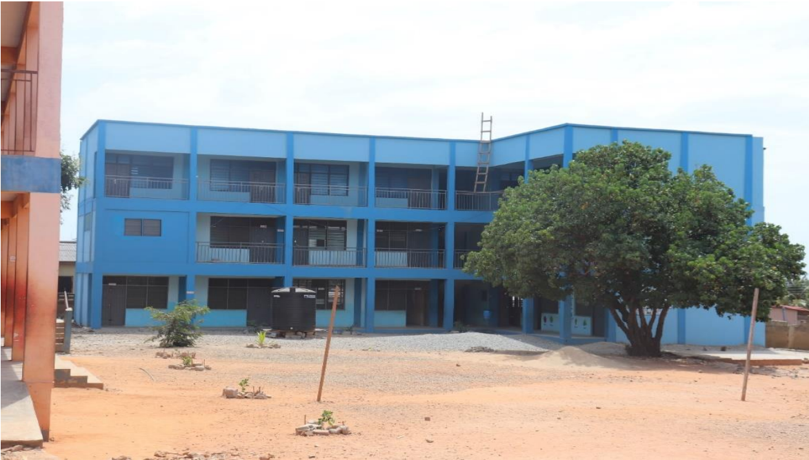
Vertical extension of 1No. 3-Storey 3-Unit Classroom Block @ Akweibu – Completed
