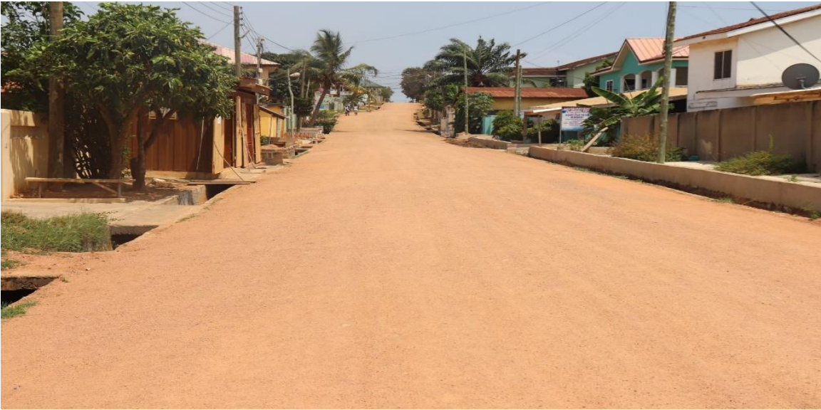
Sealing of Arko Street behind Dansoman market – 75% completed
