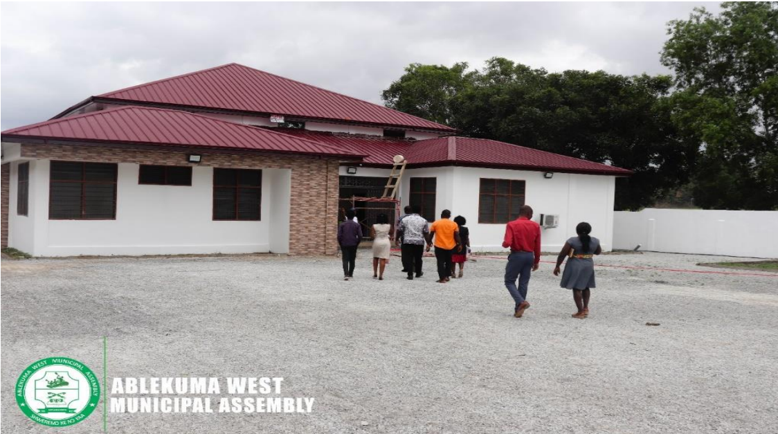
Construction of 1No. Magistrate Court @ Dansoman Keep-fit – 100% completed
