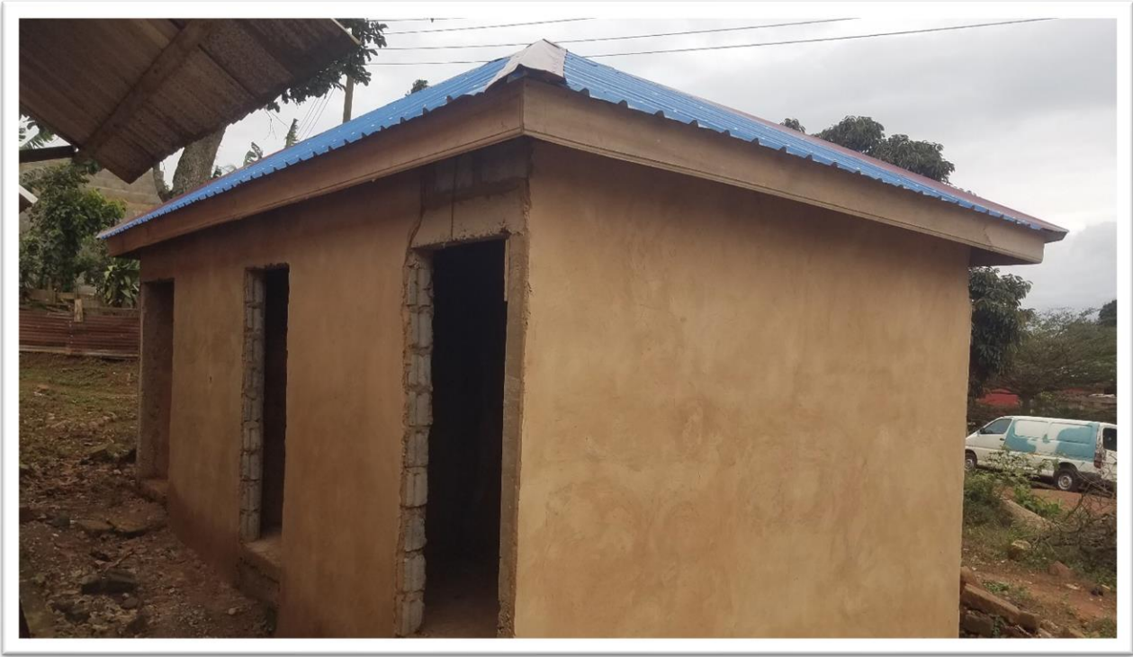
Fig 3: Toilet Facility at Adukrom Bethel JHS
