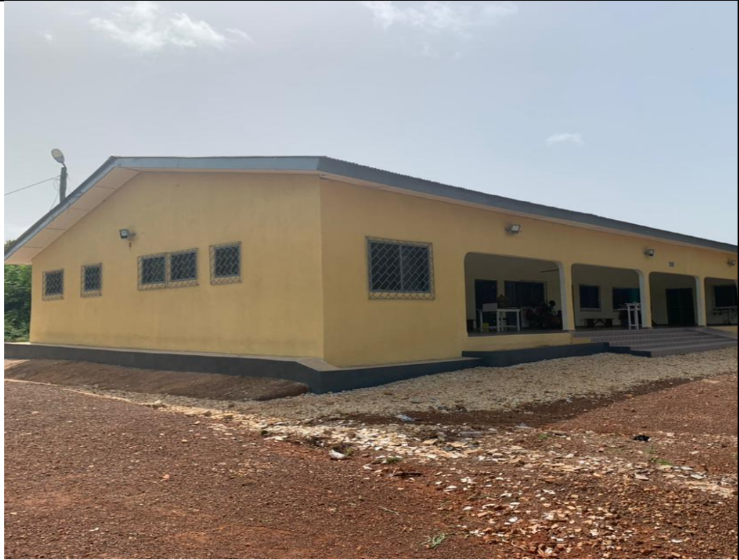
Renovated CHP's compound at Akrofufu
