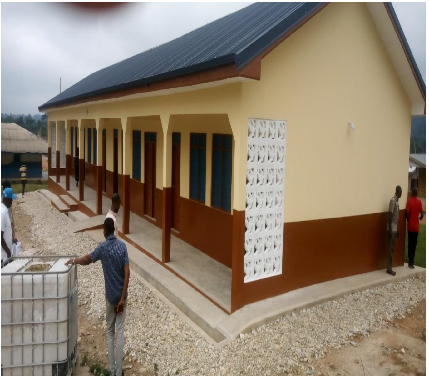
3-unit classroom block at Kadewaso
