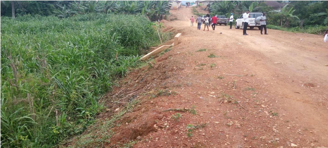
1No. Culvert at New jejeti
