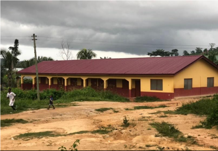
Construction of 1no. 3-unit Classroom Block at Dominase
