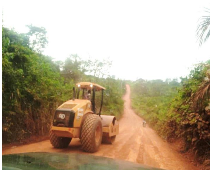
Reshaping of 30.2km feeder Roads in the District
