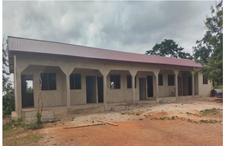
Construction of 1no. 3-unit Classroom Block at Ntom RC JHS
