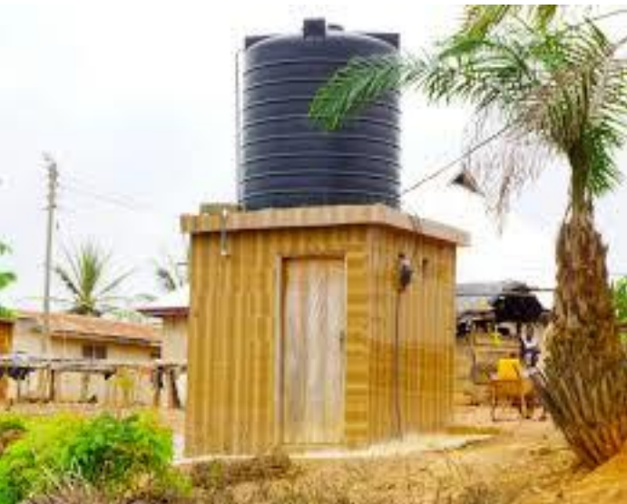
Construction of 4no. Mechanized Borehole.
