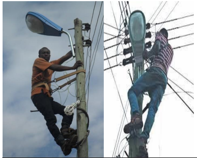
Rehabilitation of 134 Streetlights across the District
