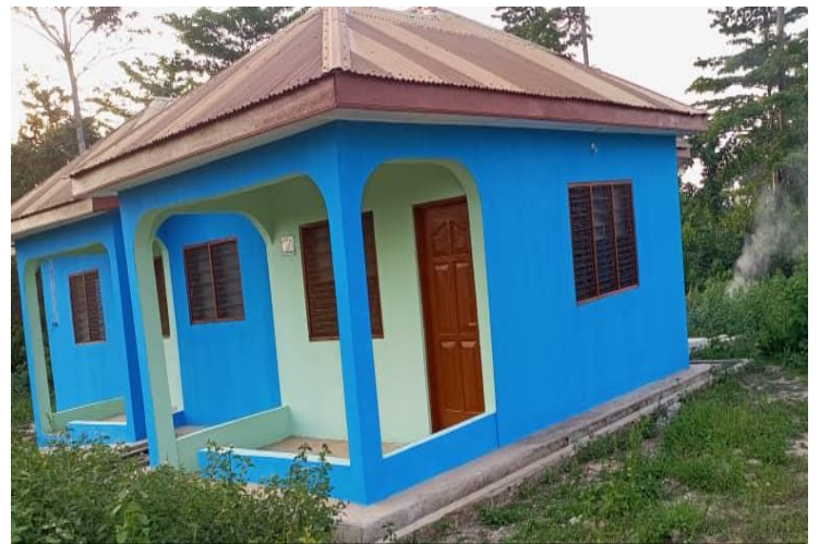
Diaso Construction of 2no. Boreholes with Renovation Works at Aburi and Besease
