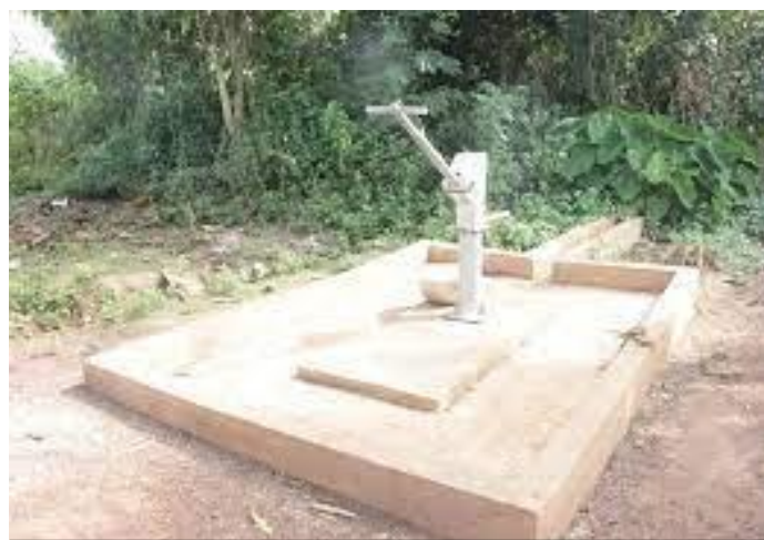
Construction of 4no. Hand Pump Boreholes
