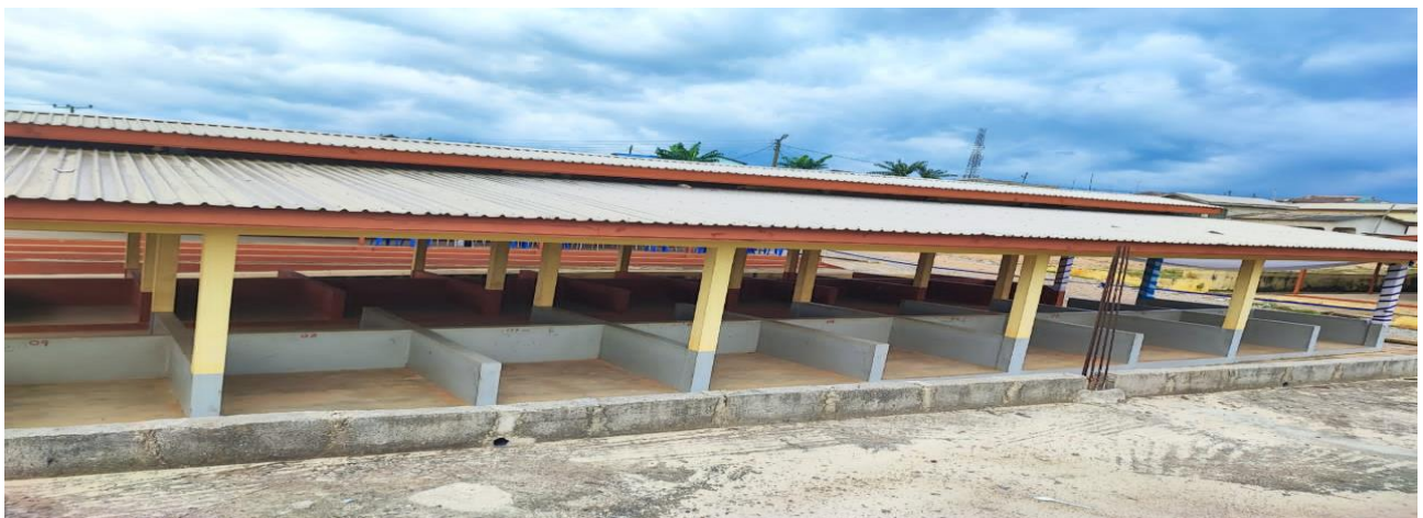
Figure 3:5 Lockable stores& 32No. Sheds at Abrem Agona
