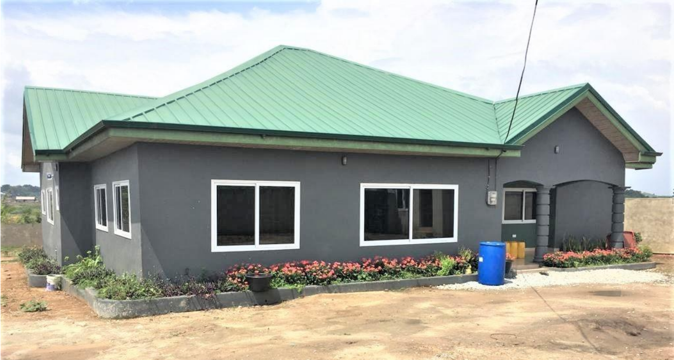
Figure 5: 1no. 3-bedroom staff accommodation Constructed at Awutu Beraku
