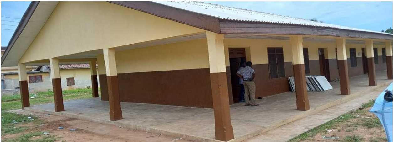
Figure 2: 1no. 3-unit classroom block Renovated at Senya
