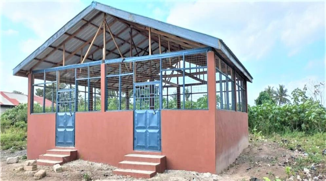
Figure 8: 1no. Cassava Processing Mill constructed at Odotom
