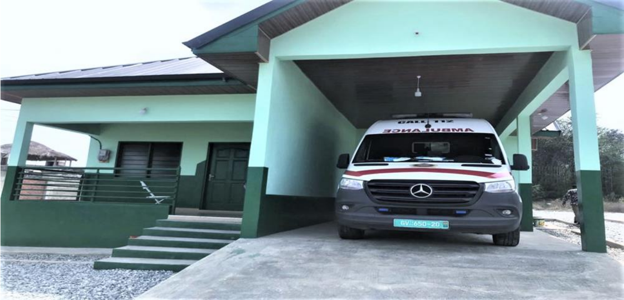
Figure 4: Ambulance bay constructed at Awutu Beraku
