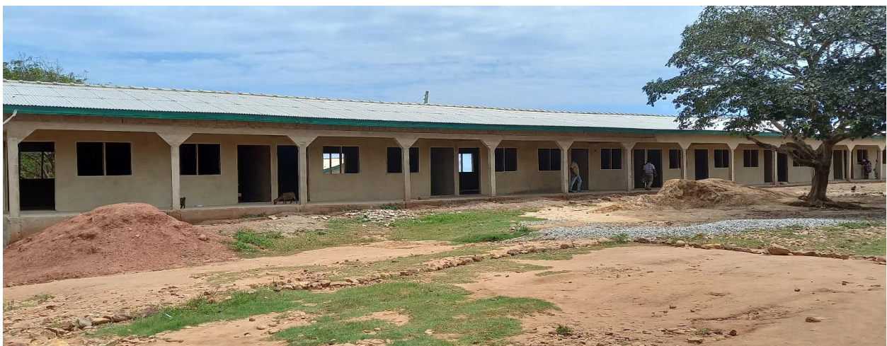
Figure 3: Construction of 6-unit classroom block at Senya (90% complete)
