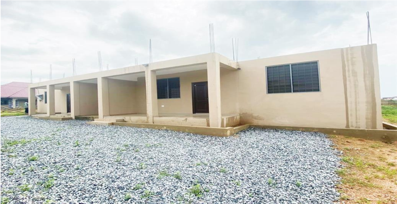
Figure 6: 1no. 2-bedroom Semi-detach Nurses Quarters Constructed at Beraku
