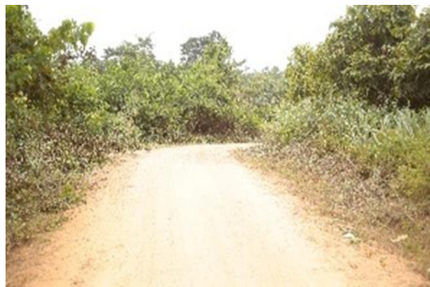
Jakai – Nyamebebu road upgraded
