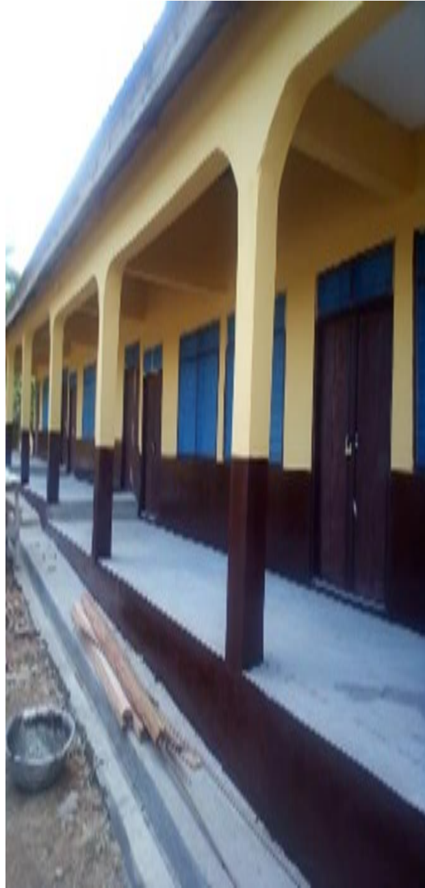
Classroom constructed at Assin Kassim
