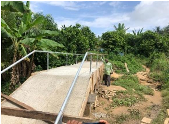
Footbridge constructed at Odumasi
