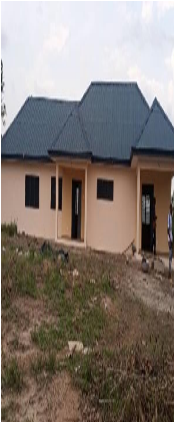
CHPS constructed at Sargentkrom
