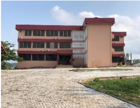
Assembly block fully renovated
