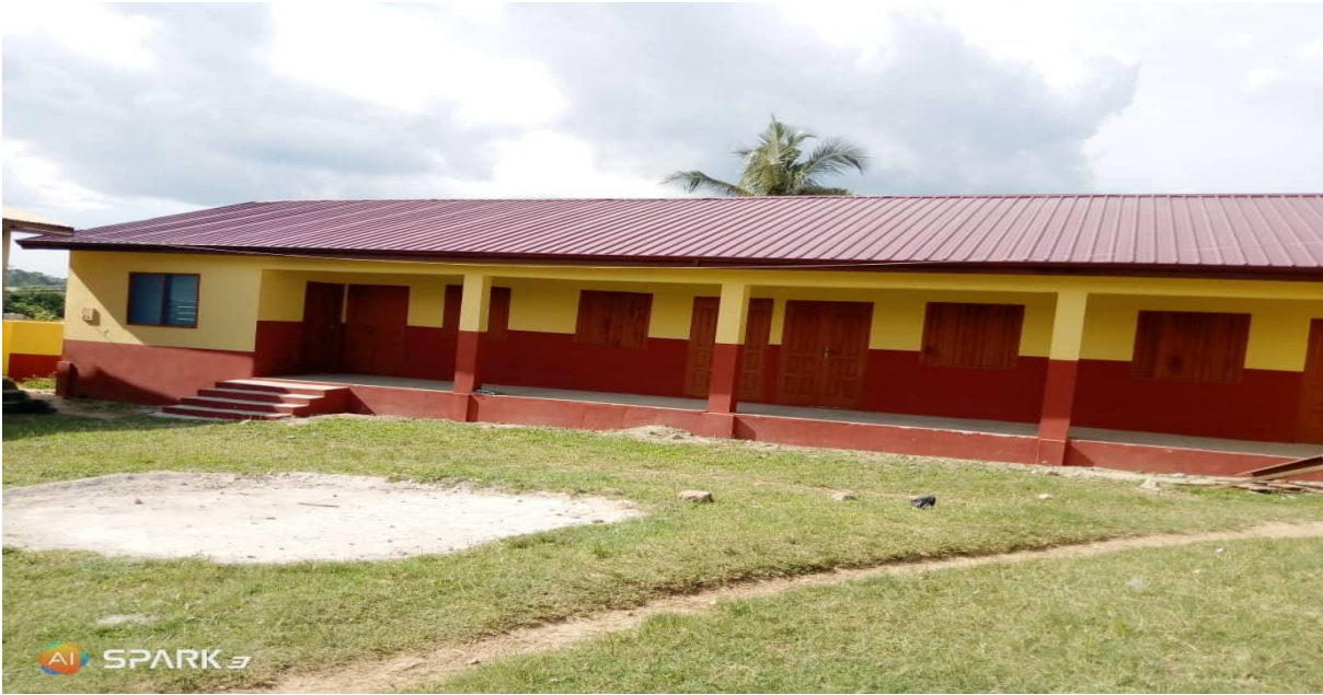
Completed and in use; 1 no. 2-units classroom block at Assin Bereku
