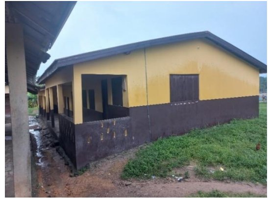
Completed 1 No 2 Unit KG Block at Breman Asikuma Methodist School
