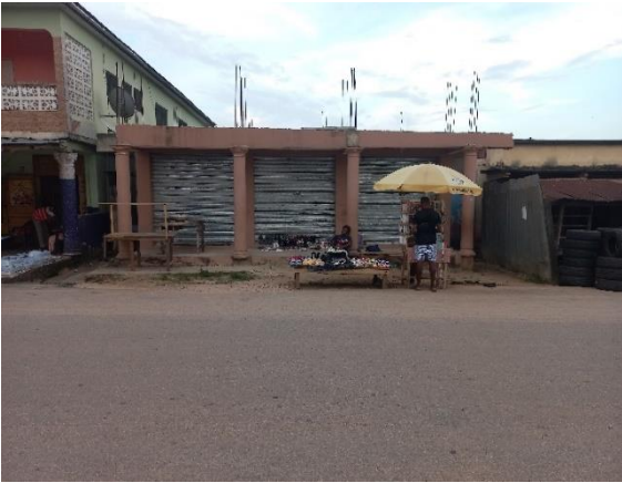
Completed 1 No. 3 Unit Trading store at Breman Asikuma Ph 1 with IGF
