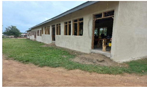
Completed 1 No. 6-Unit Classroom Block at Breman Jamra [(90% Complete)
