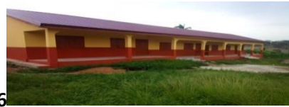
6. Completion of 1 No. 3 unit Block Classroom Block at Entumbil
