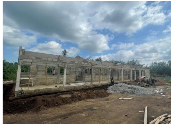
Ongoing construction of 3-unit classroom Block at Tawora
