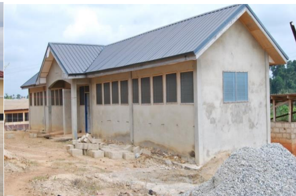
Boys Latrine at Nsaba SHS
