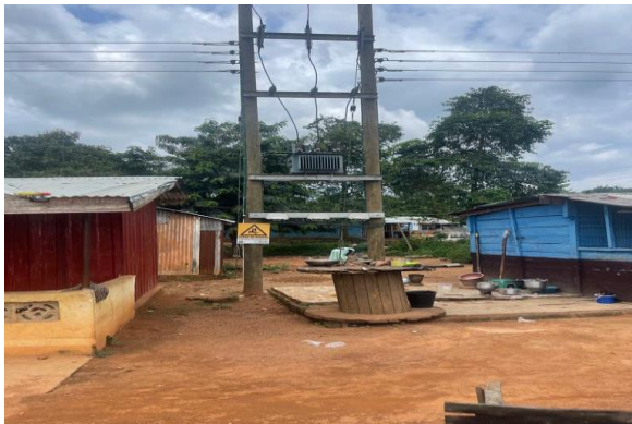
Extension of Electricity to New Communities in Duakwa
