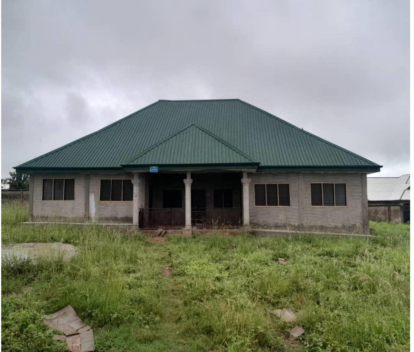
Figure 7: Constructed dressing room at the Wenchi Sports field
