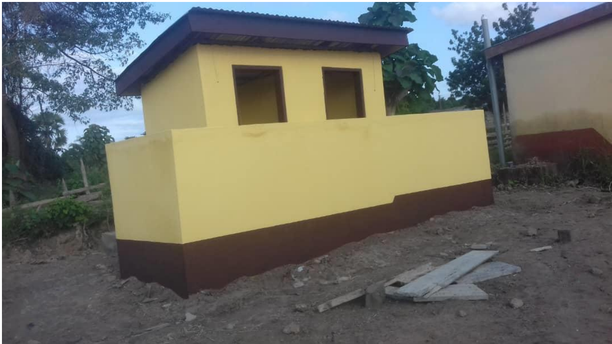
Figure 8: Constructed 2 No. 3-Unit classroom block with ancillary facilities for M/A JHS at Twumkrom/Amoakrom.
