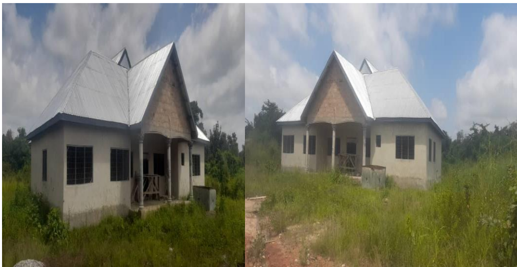
Police Post Constructed at Seikwa (Roofing and Plastering Level)
