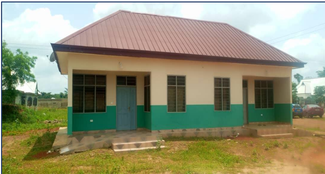
2NO. CHIPS COMPOUND CONSTRUCTED AT ATESIKROM
