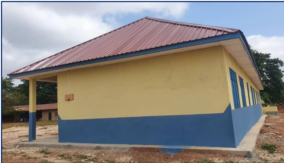
Figure 5: CONSTRUCTED 1 NO. 2 UNIT KG WITH RESTING ROOM, DINNING HALL, OFFICE AND STORE
