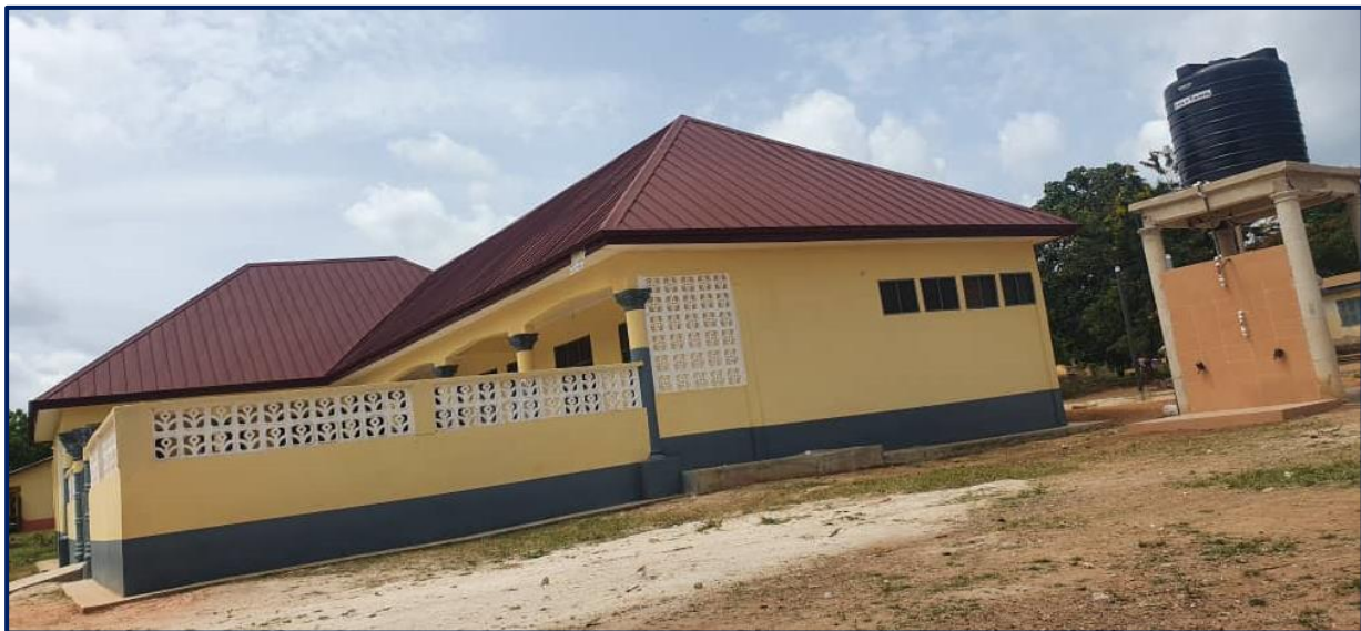
Figure 1: 1 NO. 2 UNIT KG WITH RESTING ROOM, DINING HALL OFFICE AND STORE CONSTRUCTED AT YAWKUMIKROM
