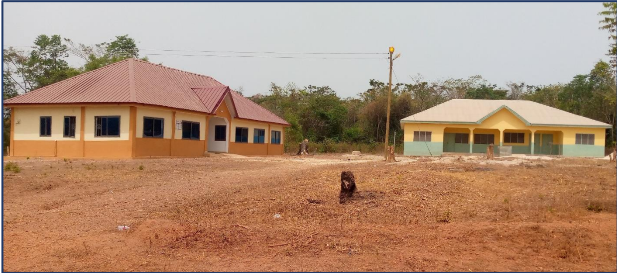
2 NO. CHIPS COMPOUND CONSTRUCTED AT MANTEWARE
