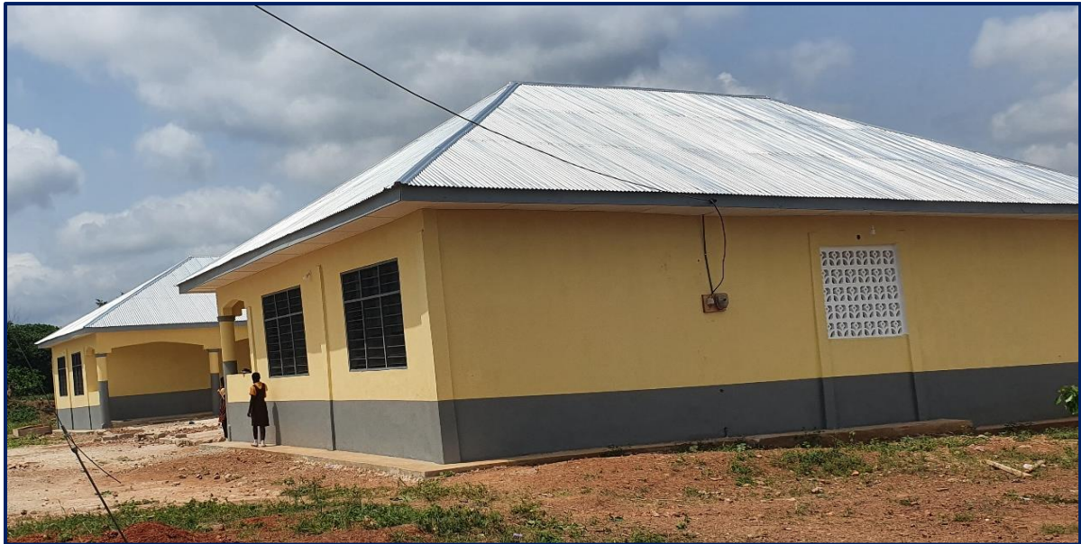
Figure 4: CONSTRUCTED 1 NO. 6 UNIT CLASSROOM BLOCK WITH OFFICE, STORE, STAFF COMMON ROOM. 1 NO. 6 SEATER KVIP & 1 NO. 2 UNIT URINAL
