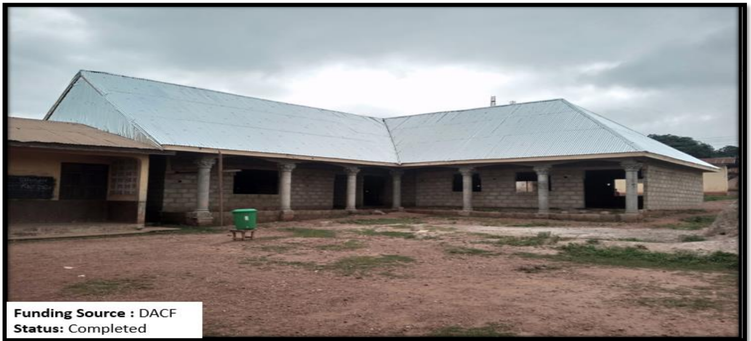
Figure 16: Roofing of SDA Primary school at Wamfie
