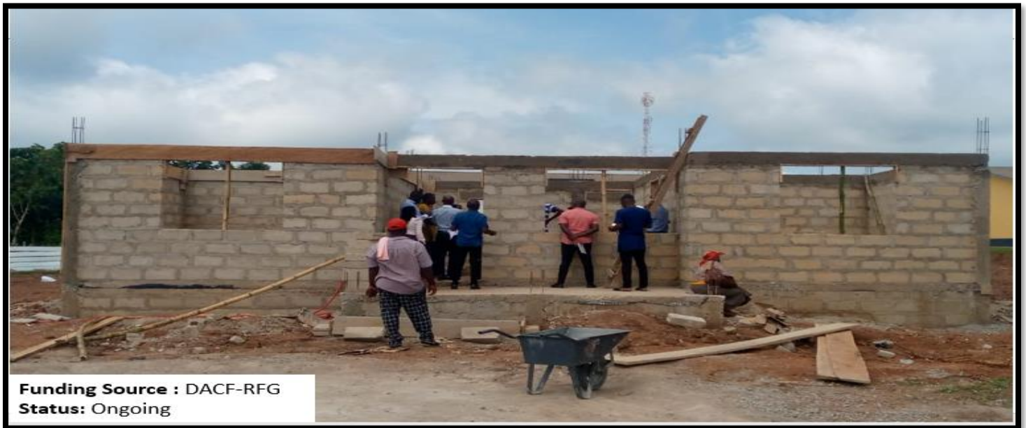
Figure 9: Construction of 1No. Staff Accommodation for GES at Wamfie
