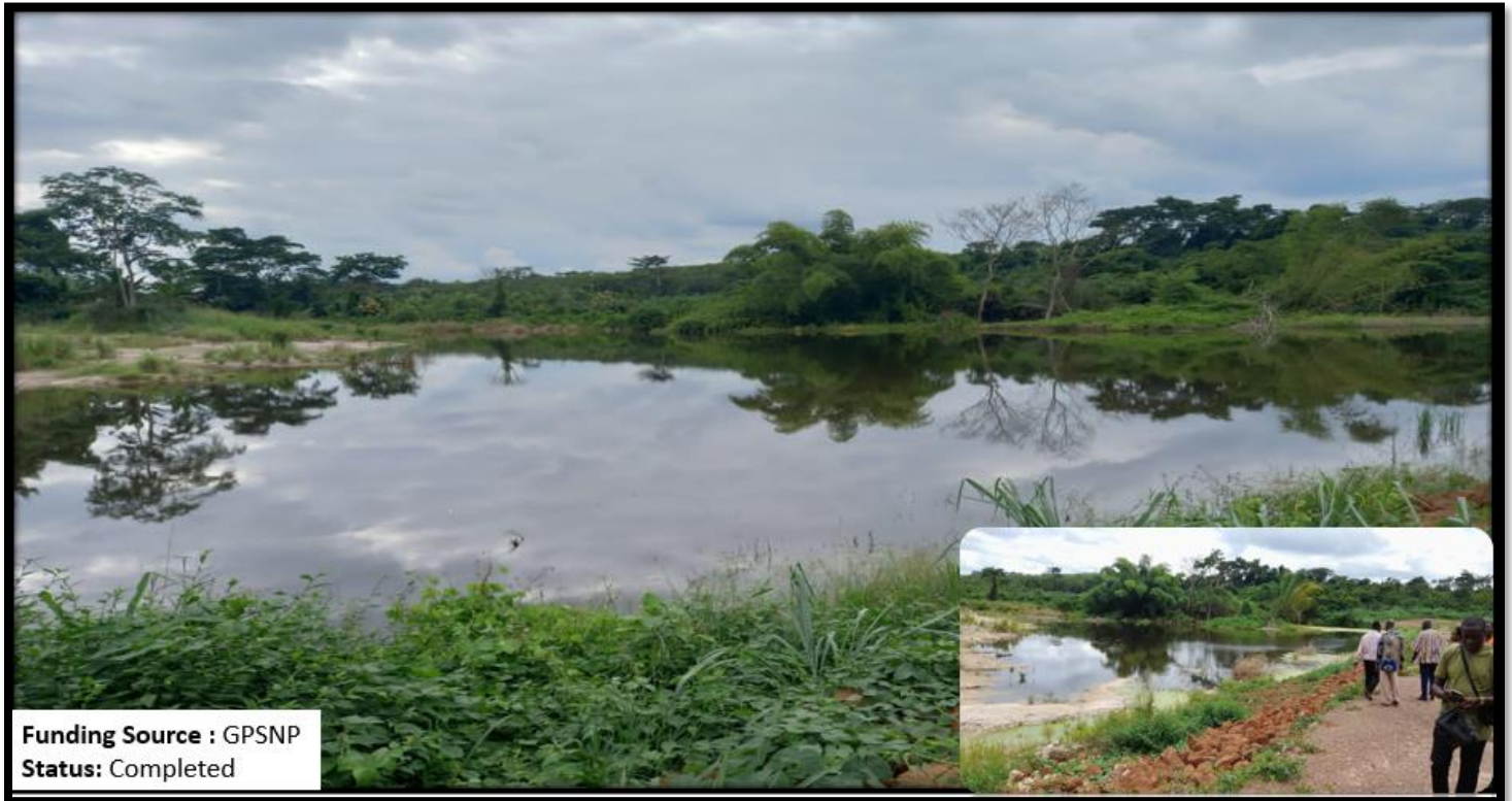
Figure 10: Rehabilitation of small Earth Dam at Nsesresu
