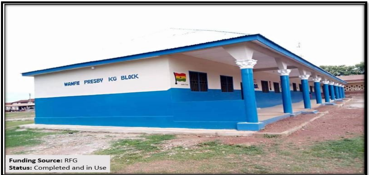
Figure 3: Construction of 4-unit classroom block at Wamfie Presby KG
