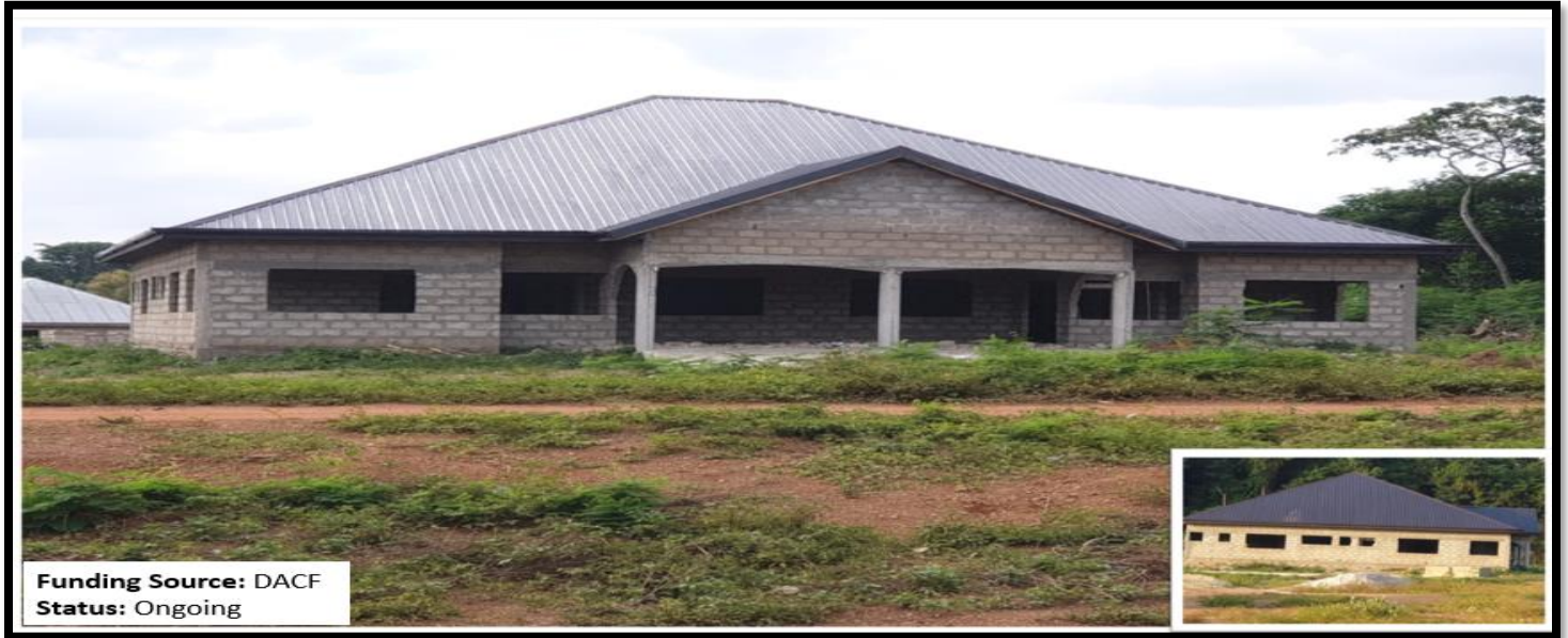
Figure 2: Construction of 1 No. CHPS Compound at Asuotiano
