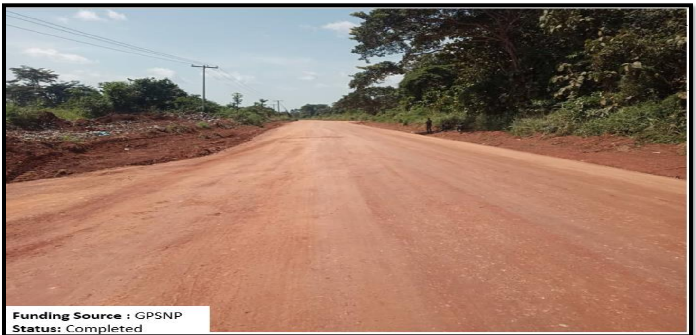
Figure 17: Rehabilitation of Kyeremasu -Kofibour feeder road (3.4km)
