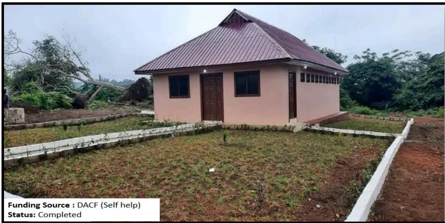
Figure 12: Completion of 1 No 20 seater toilet at Nsesresu
