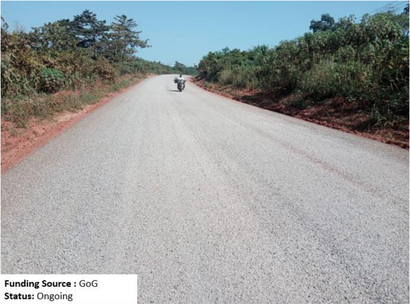
Figure 18: Upgrading of Wamfie-Adiemra (Wamfie-Sunyani) feeder road (21.20KM)
