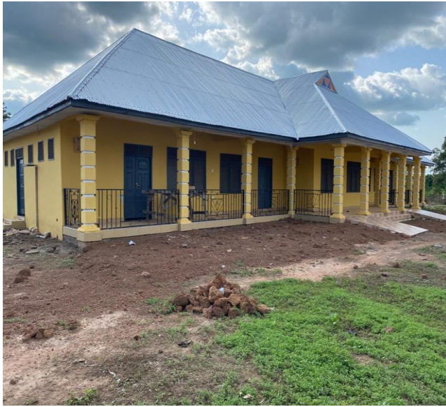
Admission ward at Abease-DACF-REG Constructed Nkwanta-DACF REG Constructed
