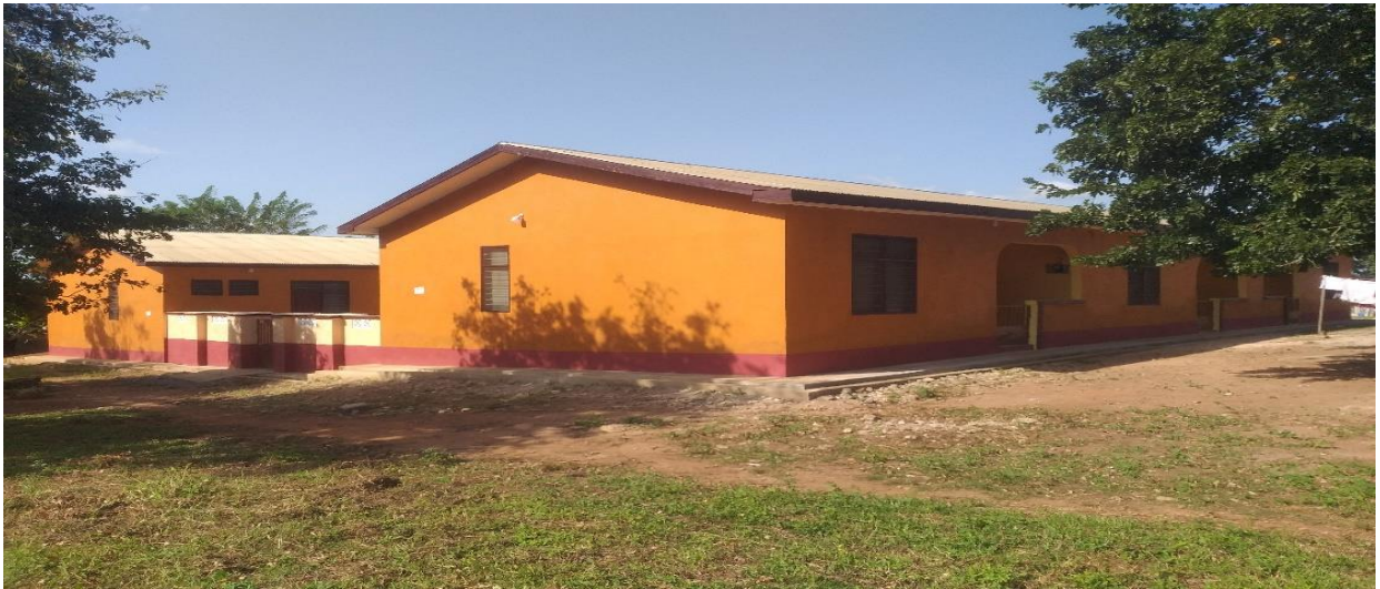
Figure 11: Renovated 1 no. 5 unit teacher's quarter at Beposo- DCAF
