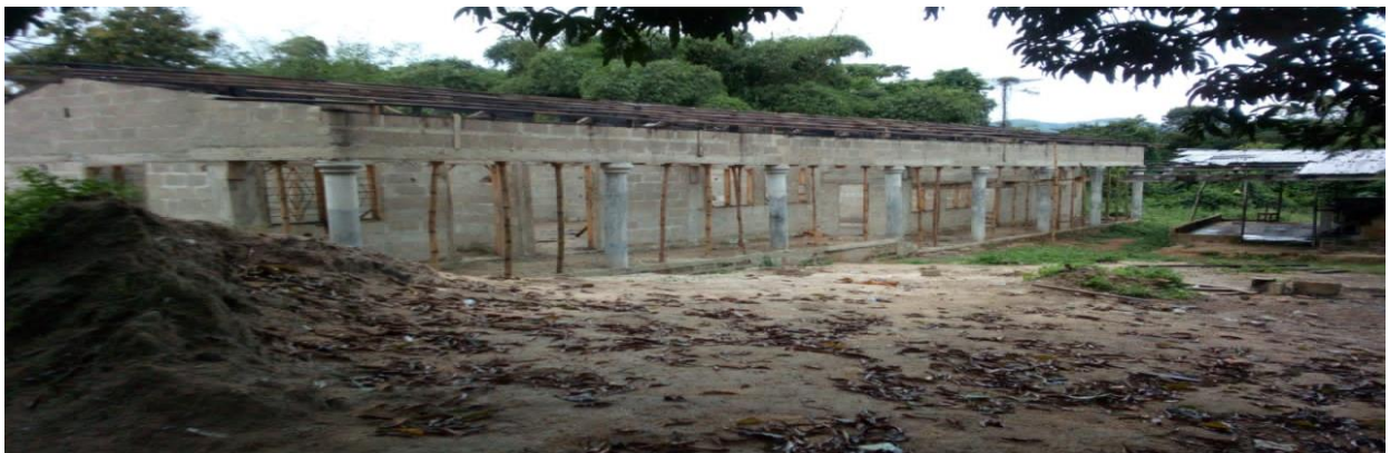
Figure 8: Construction of 1no. 3-unit classroom block at Adutwamu – DACF-RFG
