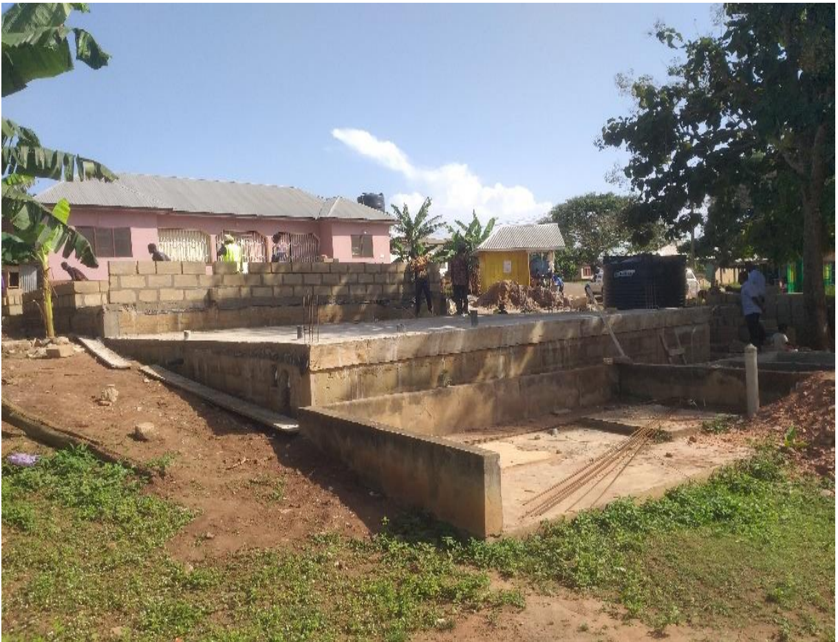
Figure 12: Construction of 1 no. 3 unit self-contained Nurses quarters at Beposo. –DCAF-RFG
