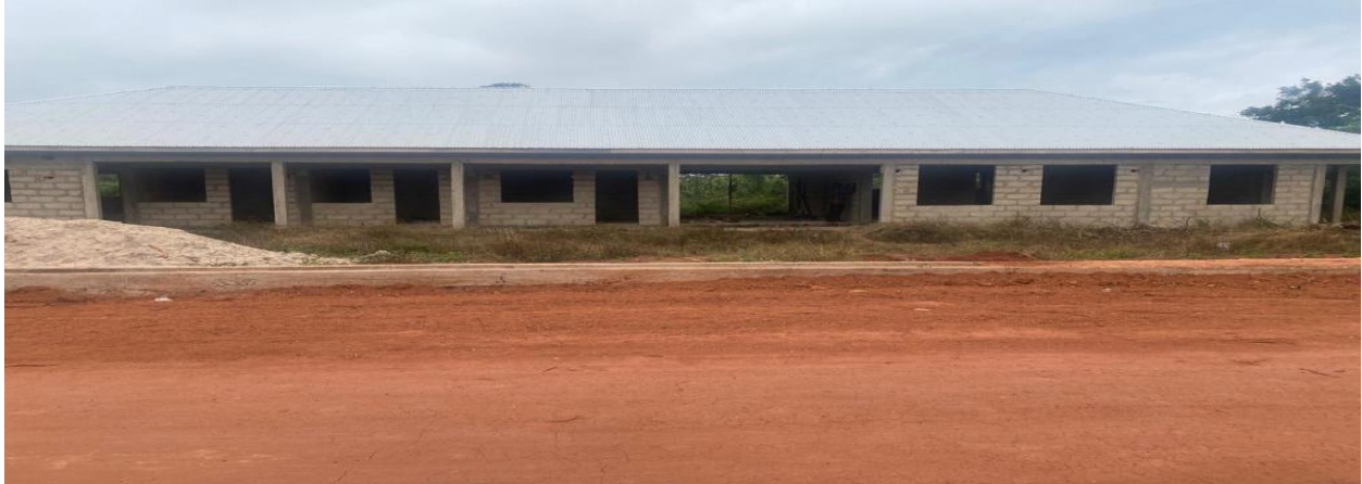
Figure 6: Construction of Agric veterinary office at Kwamang-DACF-RFG
