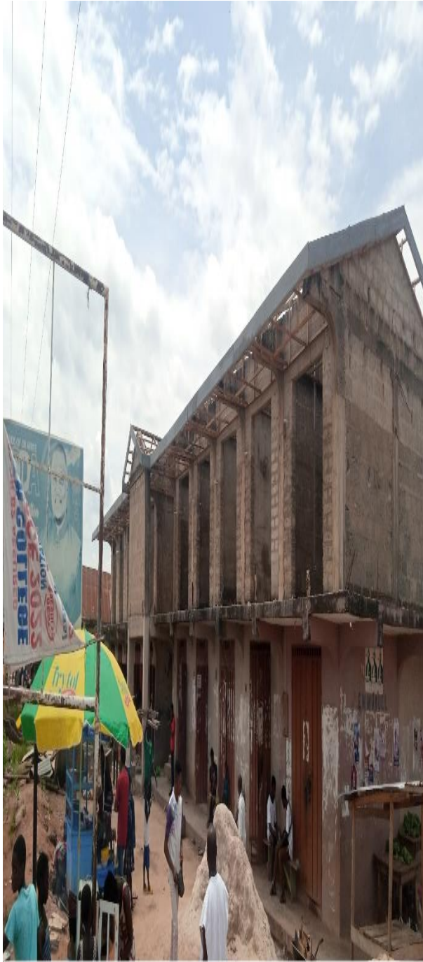
DACF-RFG REHABILITATION OF 40 LOCKABLE STORES AT ASOKORE AR-0022-2681
