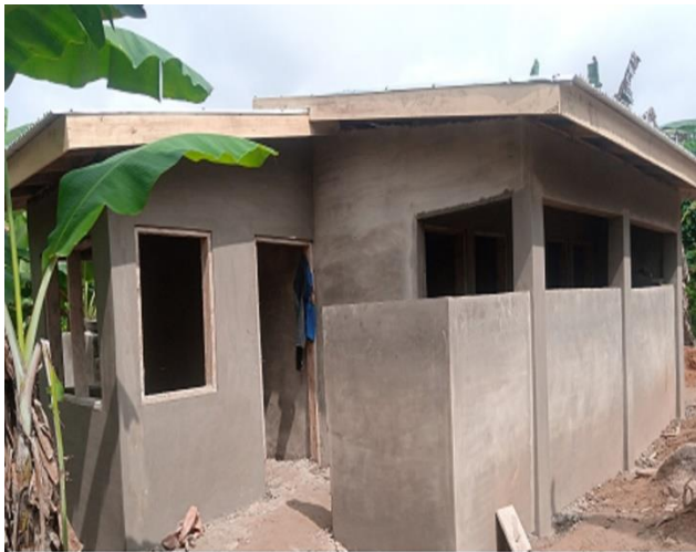
1 No. 10 Aqua Seater Toilet At Akwakrom GPS: AR-0472-6548, Founding Source: DACF/RFG
