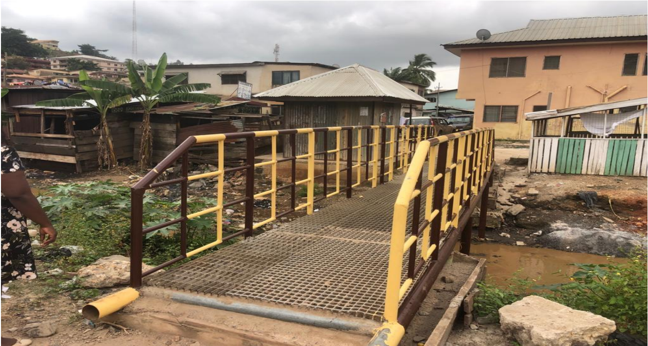
FOOTBRIDGE CONSTRUCTED AT TUTUKA KWABRAFOSO
