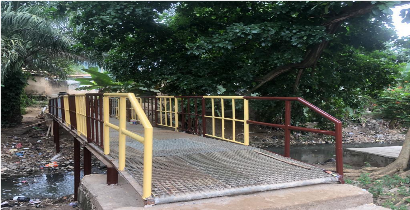
Footbridge constructed at aboagyekrom
