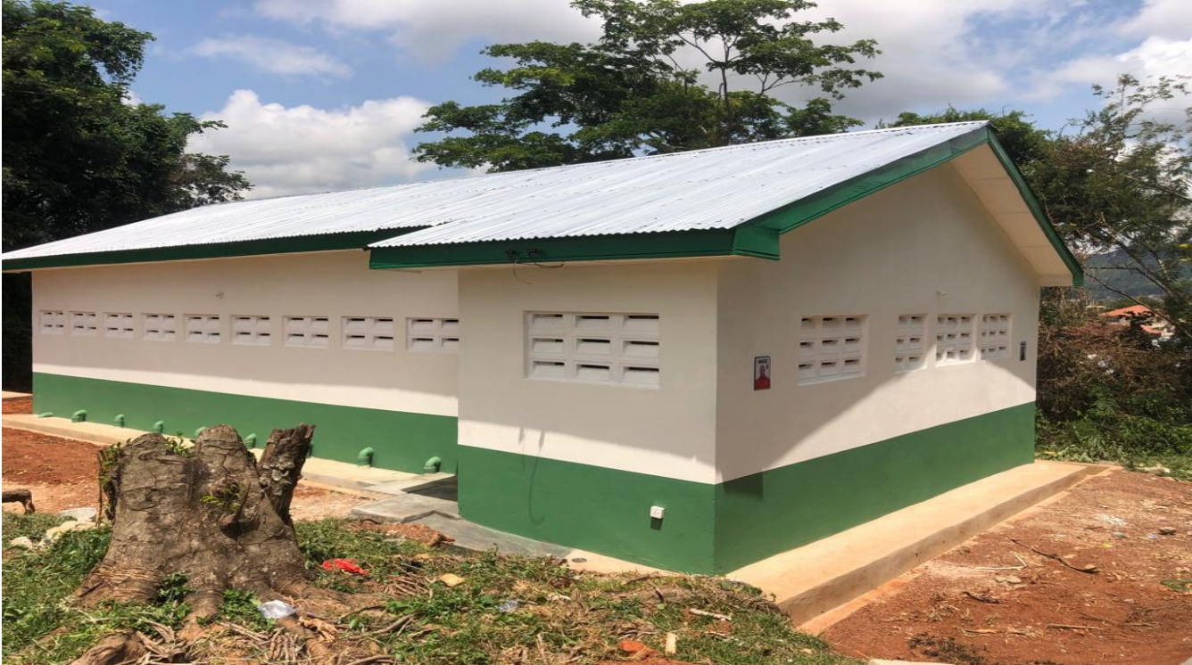
Constructed Toilet facility at CKC Senior High School
