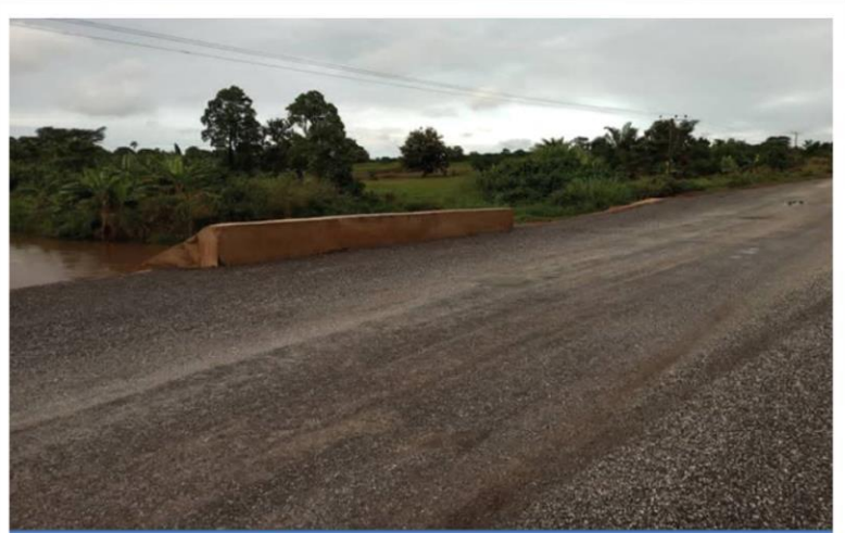
PROJECT DESCRIPTION: CONSTRUCTION OF ATONSUAGYA ROAD DIGITAL ADDRESS: AM-2553-2368
