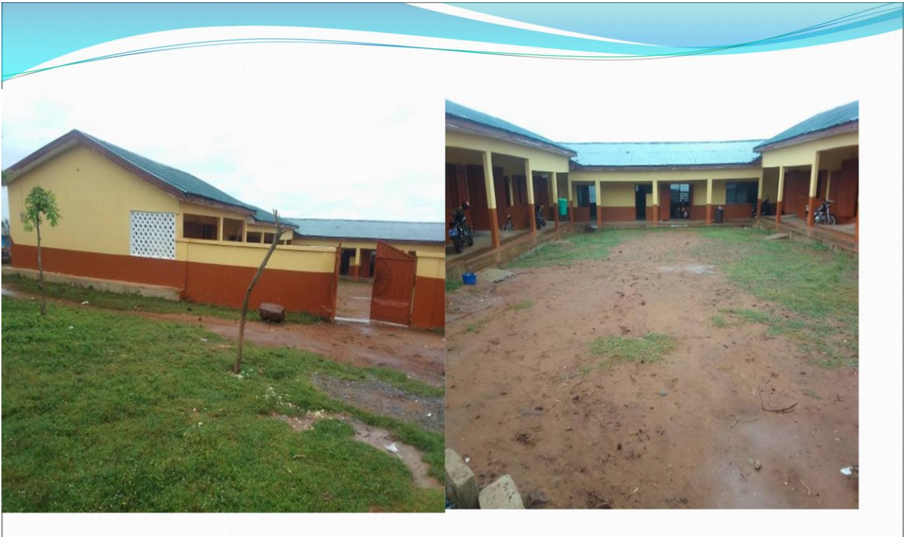
CONSTRUCTED 1NO.6UNIT CLASSROOM BLOCK AT NYAMEBEKYERE
