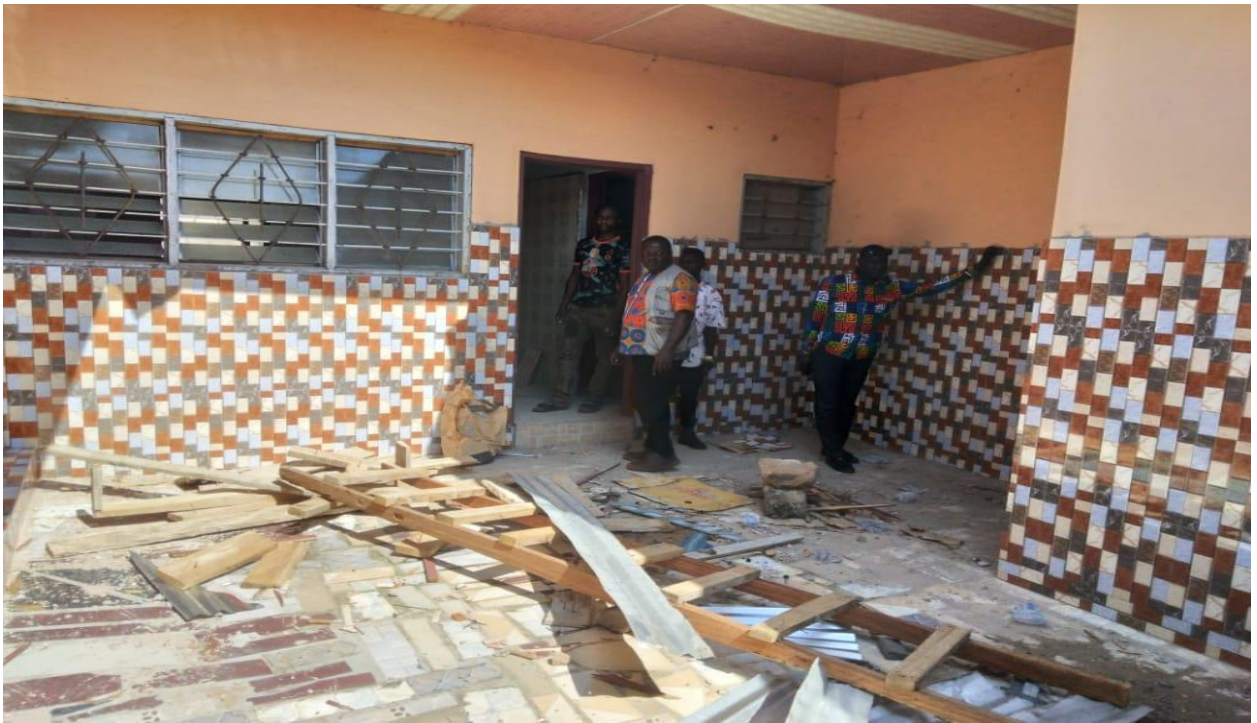
RENOVATED MCE'S RESIDENCE
