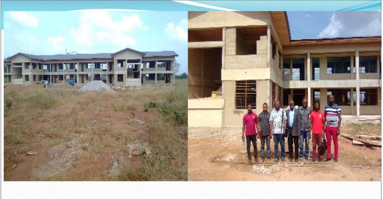
CONSTRUCTED 1NO.1STOREY 24UNIT CLASSROOM BLOCK AT AWOBA SHS-ANYINASU
