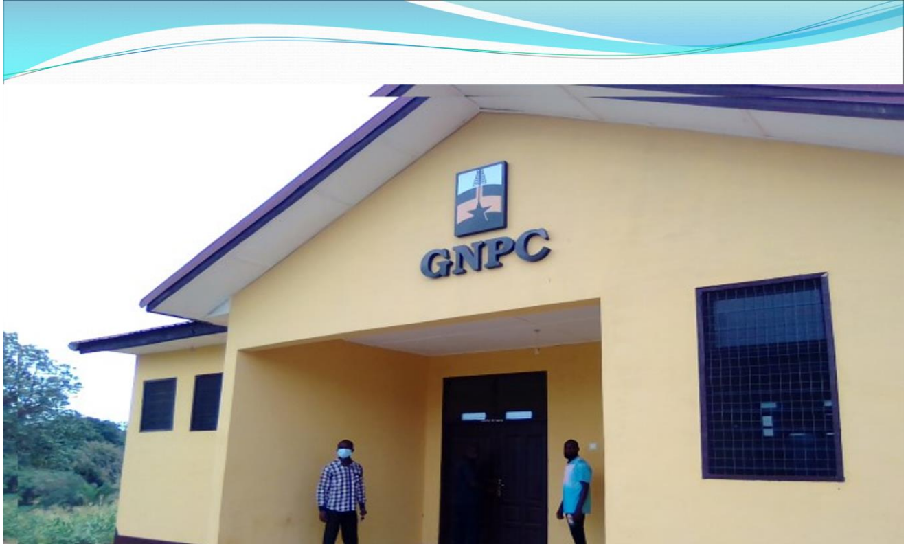
CONSTRUCTED 10 SEATER WC TOILET AT EJURAMAN SENIOR HIGH SCHOOL
