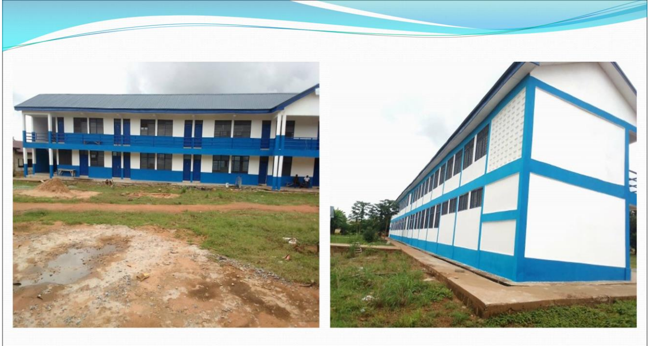
CONSTRUCTED 1-STOREY GIRLS DOMITORY AT EJURAMAN SENIOR HIGH SCHOOL
