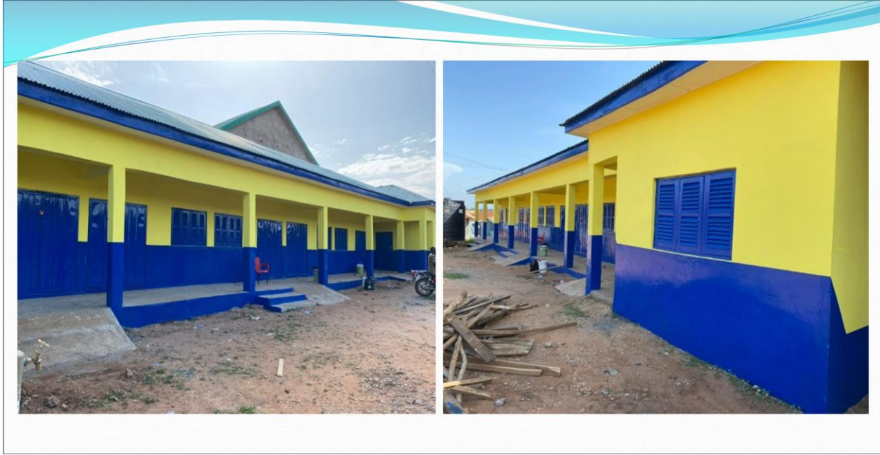
CONSTRUCTED 1NO.3UNIT CLASSROOM BLOCK AT EJURA METHODIST
