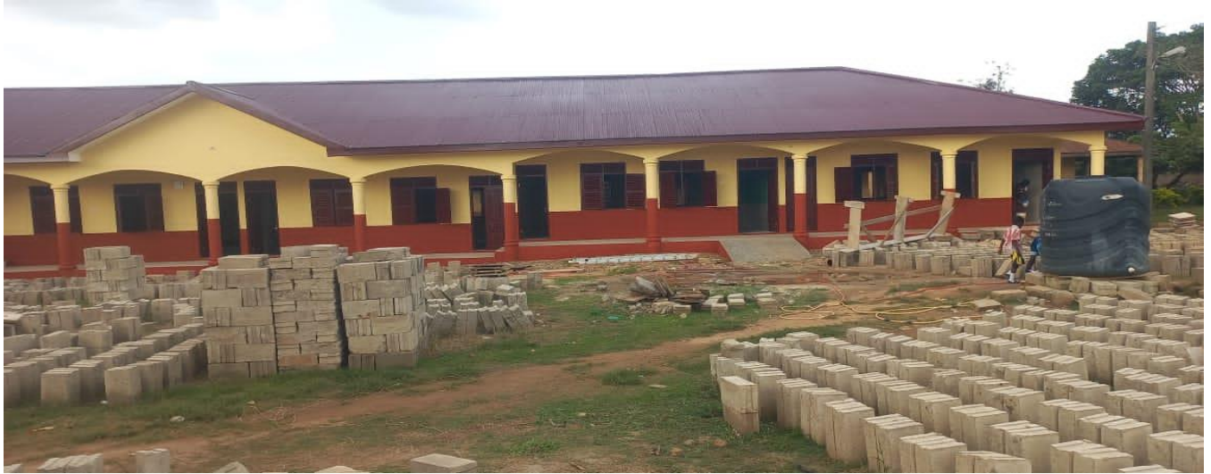
1No. 6-unit classroom block with office, store, 6-seater WC toilet completed at Achinakrom
