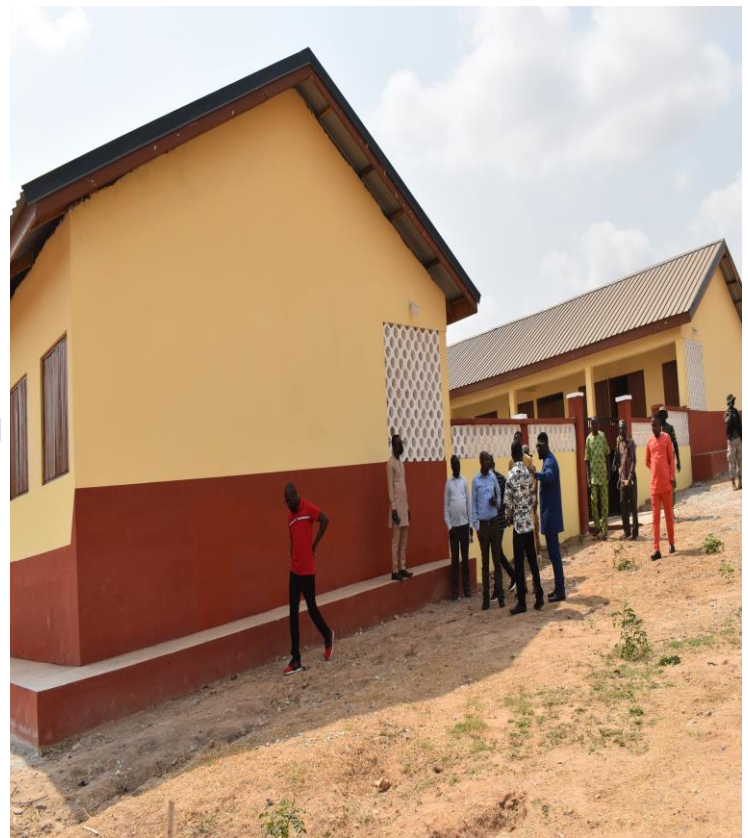
AFRANCHO CLASSROOM BLOCK
