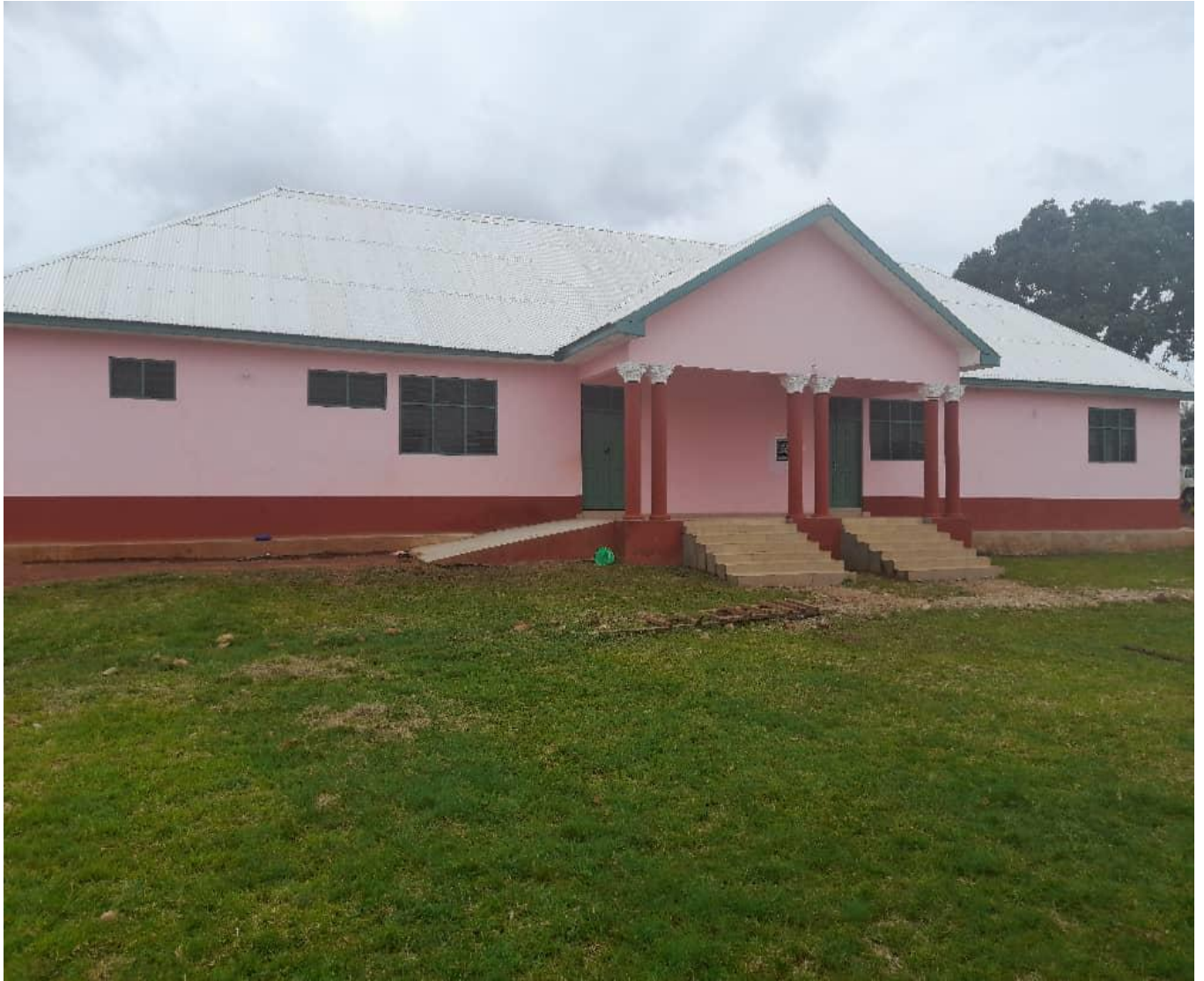
Completed dormitory for Boakye Tromo SHTS @ Ghc 293,641.68 (DACF-RFG)
