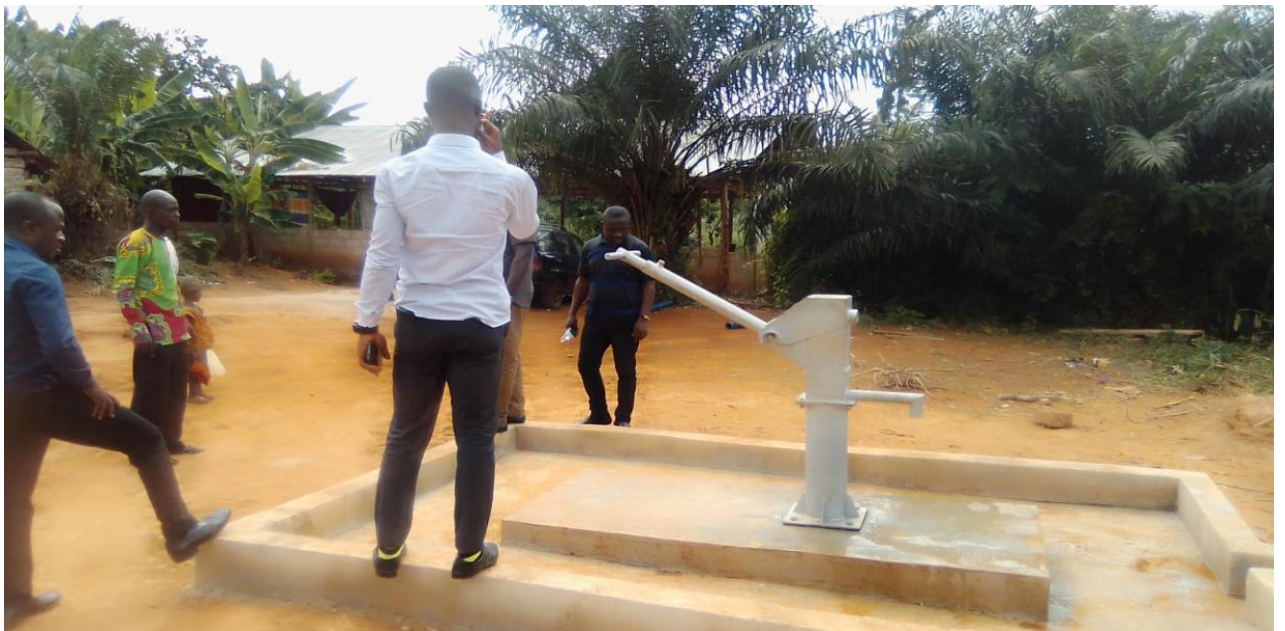
4 No. Boreholes, Location: Atudrubesa, Yaw Nyarko, Nkwadwofobehu and Mpensembi @ Ghs139,981.96 (DACF-RFG)
