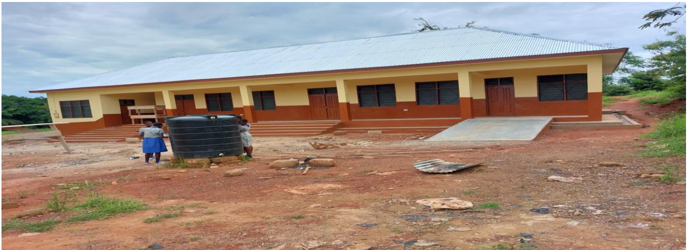
1NO. 3-Unit Classroom Block at Tanoso SDA Primary School, Funding: GRC
