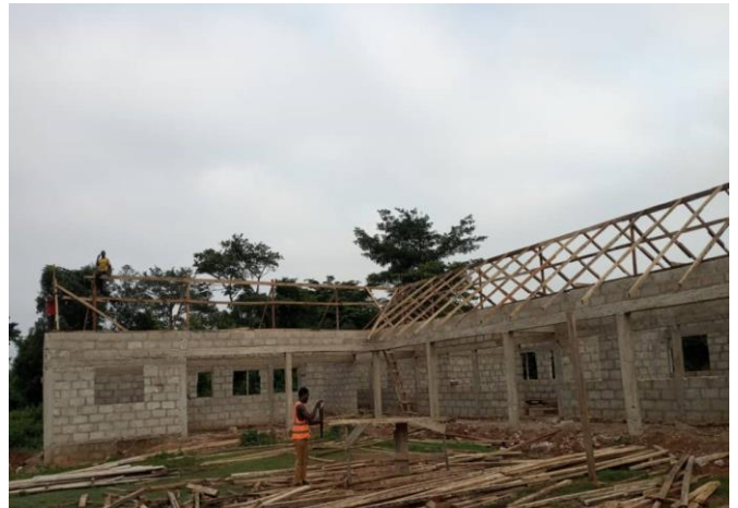
☐ 1NO. 3-UNIT CLASSROOM BLOCK AT DONKORK 1
