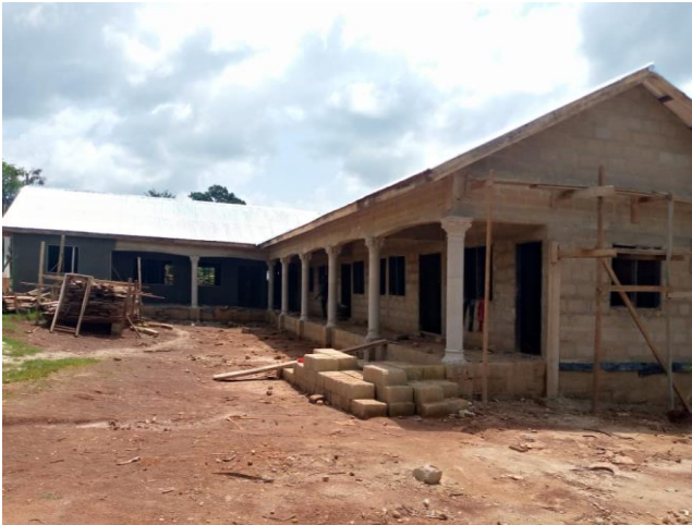
☐ 1NO. 3-UNIT CLASSROOM BLOCK AT DONKORK
