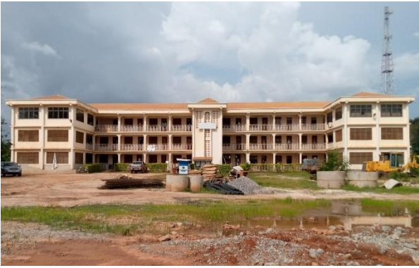
REHABILITATION OF THE DISTRICT ASSEMBLY
