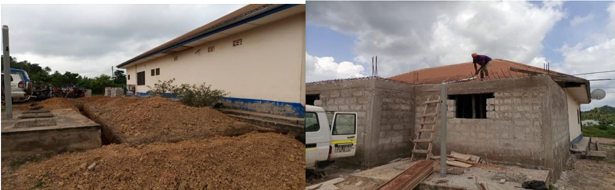
10. Construction of 1no. 2-Unit Cell at Aboso Police Station
