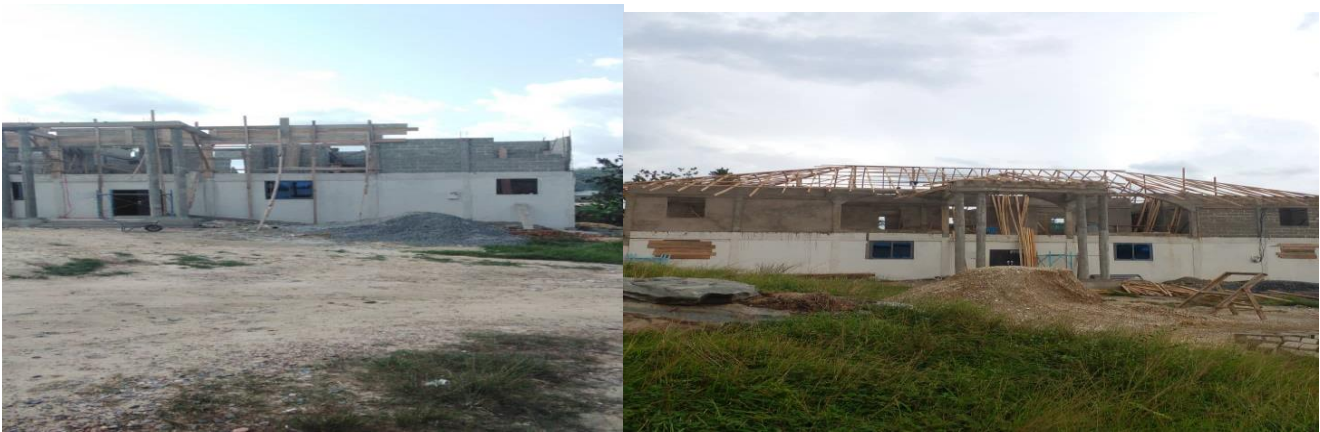
11. Completion of 1no. ICT Centre Tt M.A School, Bogoso
