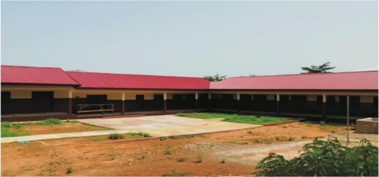
CONSTRUCTED 1 NO. 6 UNIT CLASSROOM BLOCK @ BRADA TORNU
