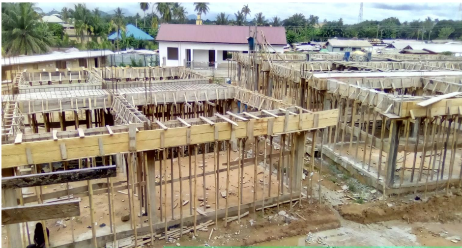
Construction of 144 market stalls at Hohoe market on- going project
