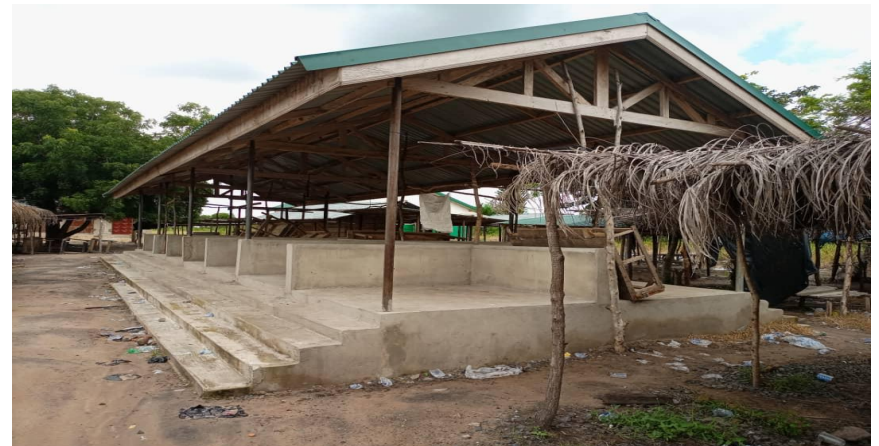
Constructed 1No. 14-unit market sheds at Animal Market –
