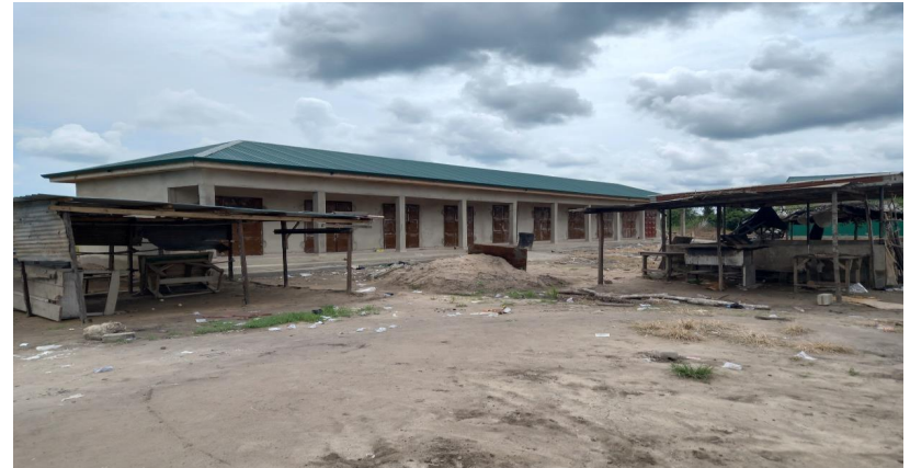
Constructed 1No. 10-unit lockable stores at Animal Market
