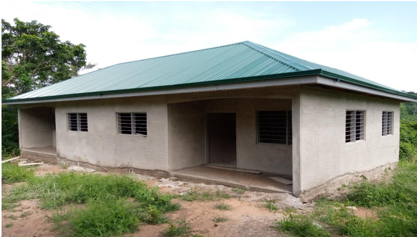
Constructed Nurses quarters at Adaklu Kordiabe
