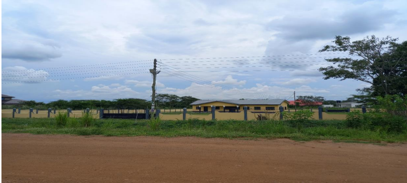
Constructed fence wall at Waya District Police Headquarters
