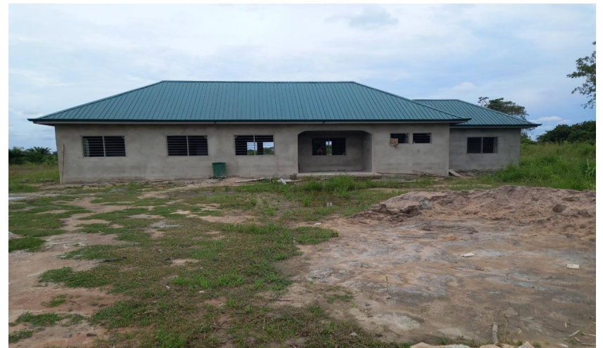
Constructed Adaklu Ablornu Health Centre with ancillary facilities
