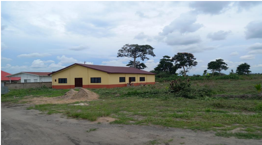
Constructed District Police Canteen at Waya
