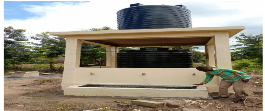
Drilled of 1No. mechanized borehole at Adaklu Abuadi
