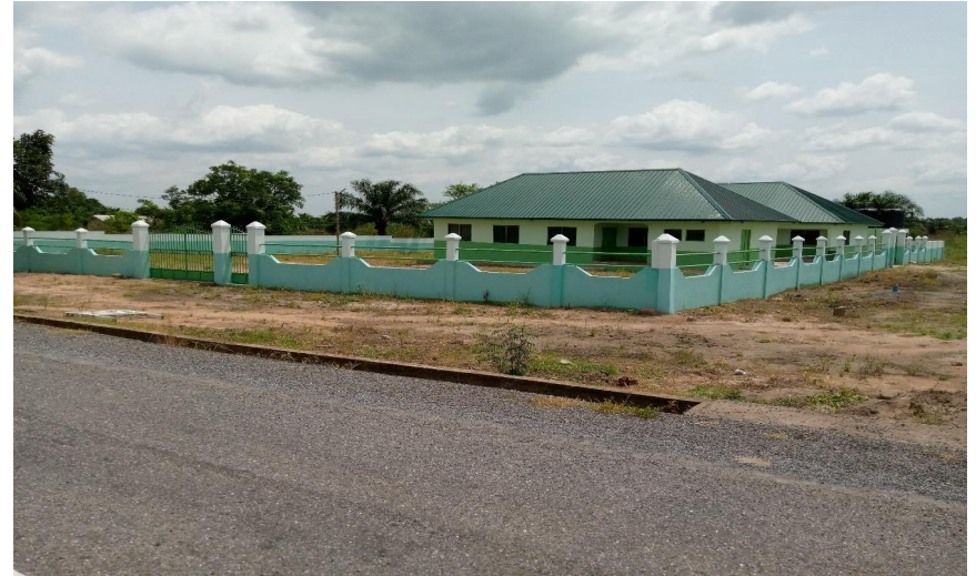
Constructed fence wall at Anfoe CHPS Compound
