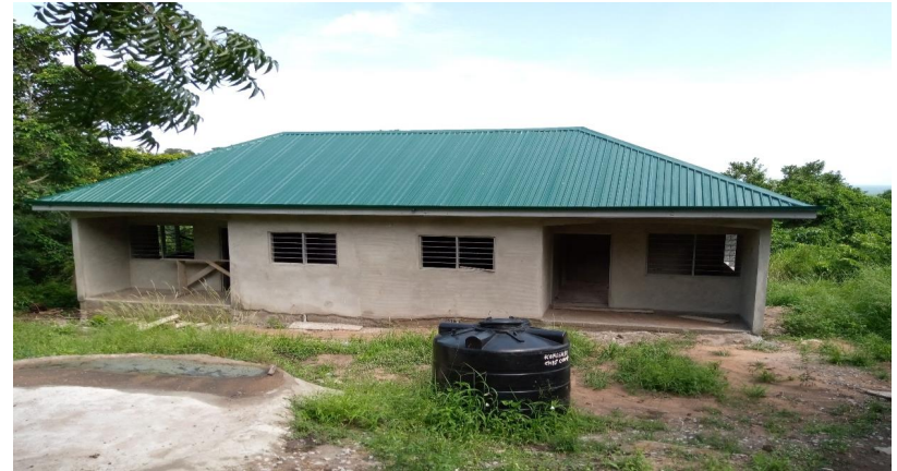
Constructed Nurses quarters at Adaklu Hlihave
