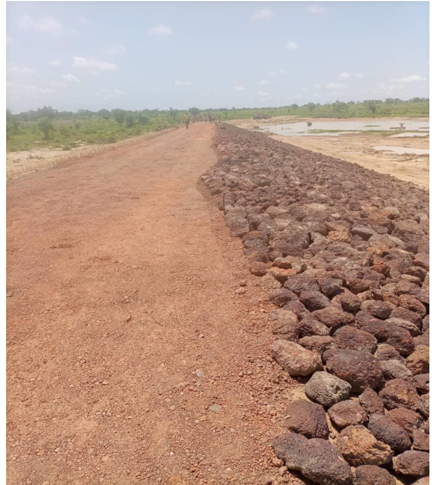
CONSTRUCTION OF SMALL EARTH DAM AT BERWONG
