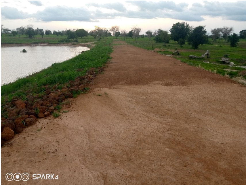
CONSTRUCTION OF SMALL EARTH DAM AT YAGRA
