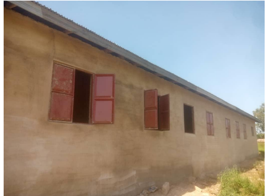
CONSTRUCT 1NO. 3-UNIT CLASSROOM BLOCK AT TAMPIE
