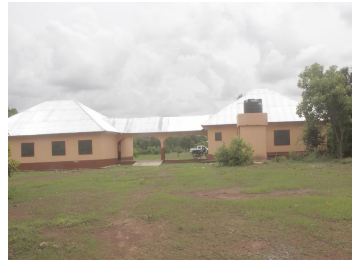
Construction of CHPS Compound at Gunwagré under DACF
