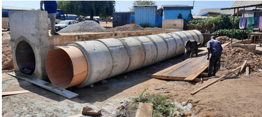
Constructed 2no. Box Culverts (DACF-RFG)
