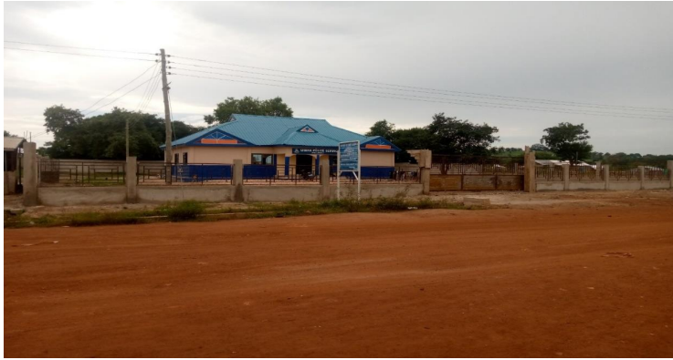
Constructed 1No. disability friendly District Health Administration office block with ancillary facilities at Garu (DACF-RFG)
