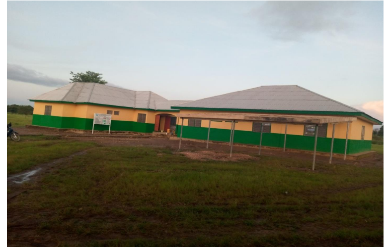
Construction of CHPS Compound at Gane-Asongé under DACF
