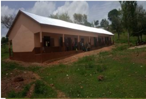
Construction of 3-Unit Classroom Block at Damolgu Primary School under
