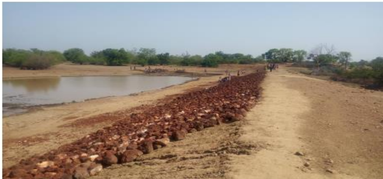
BUILSA SOUTH DISTRICT, FUMBISI
