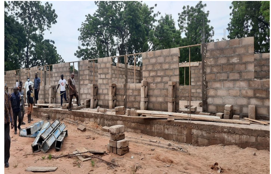
Construction of 3-Unit classroom Block with Ancillary Facilities at Kansoe
