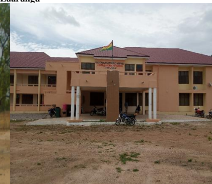
Constructed District Assembly complex in Zuarungu
