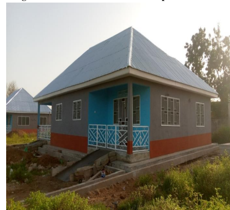
Constructed of 2no. 2-Unit Semi-detached bungalows for staff of decentralized departments
