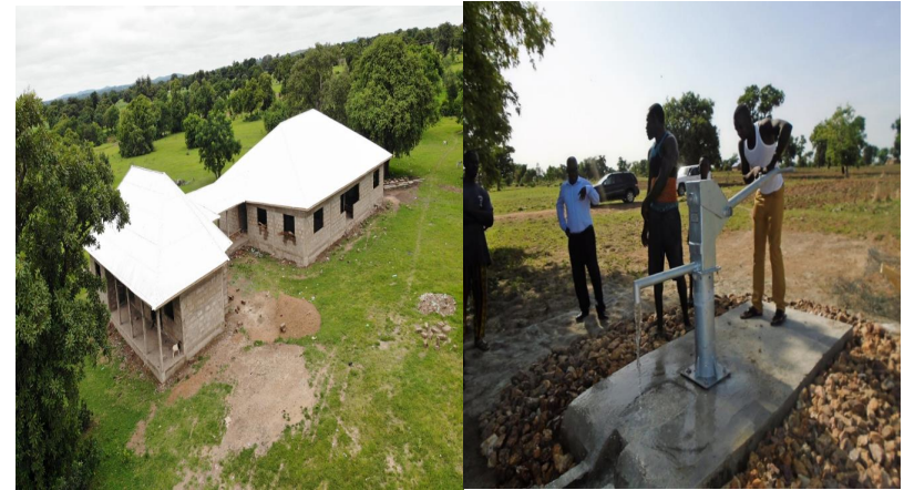
Construction of 1no. CHPS at Kunkua-Asonge Constructed 83no. boreholes district-wide
