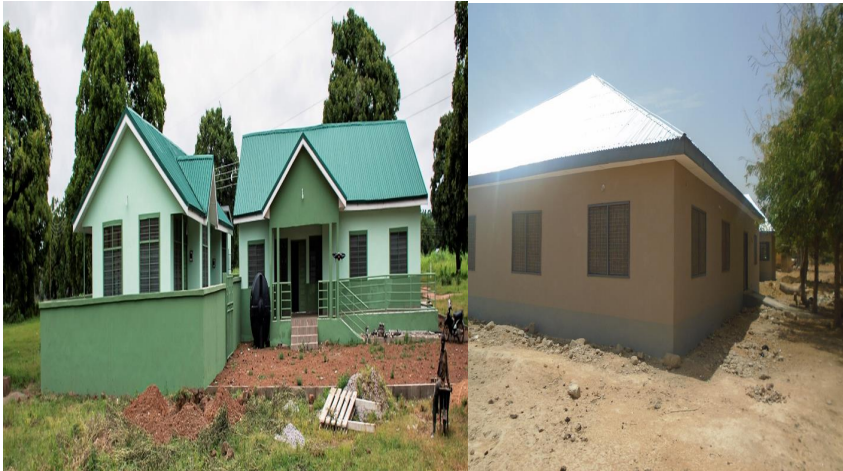
Constructed 2no. CHPS Compounds at Sakaribisi and Zuarungu-Moshie
