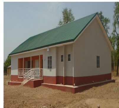
Constructed 1no. District Magistrate Court
