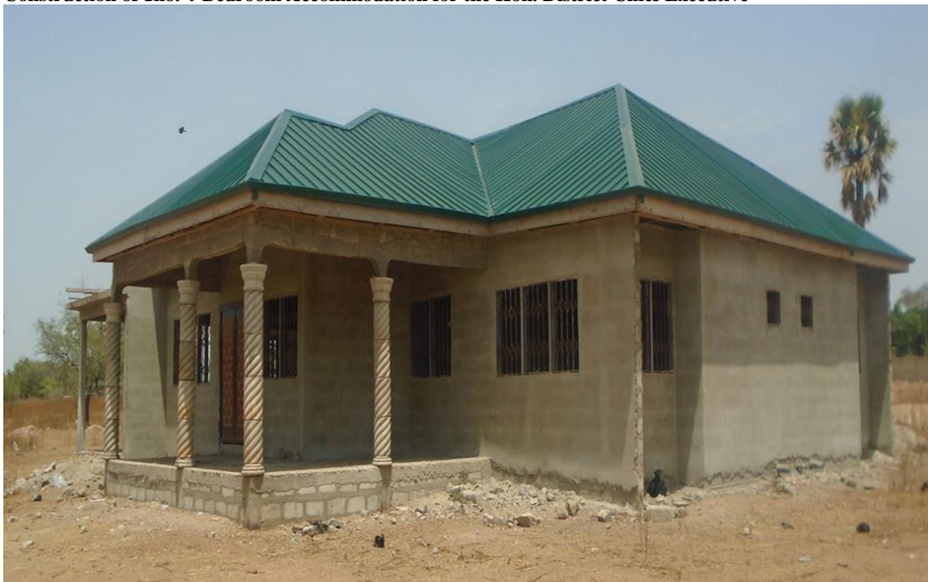
Construction of 1no. 4-Bedroom Accommodation for the Hon. District Chief Executive
