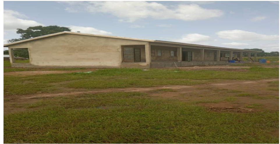
3-Unit classroom block at Shega constructed
