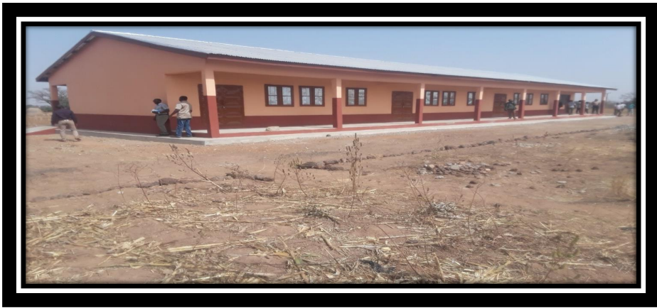
3-Unit classroom block at Asapalugu constructed
