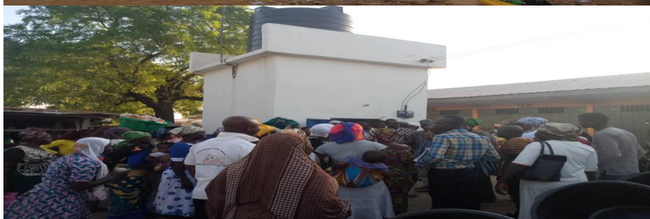
3No. Covid-19 water systems at Zebilla,Binaba and Sepeliga township constructed
