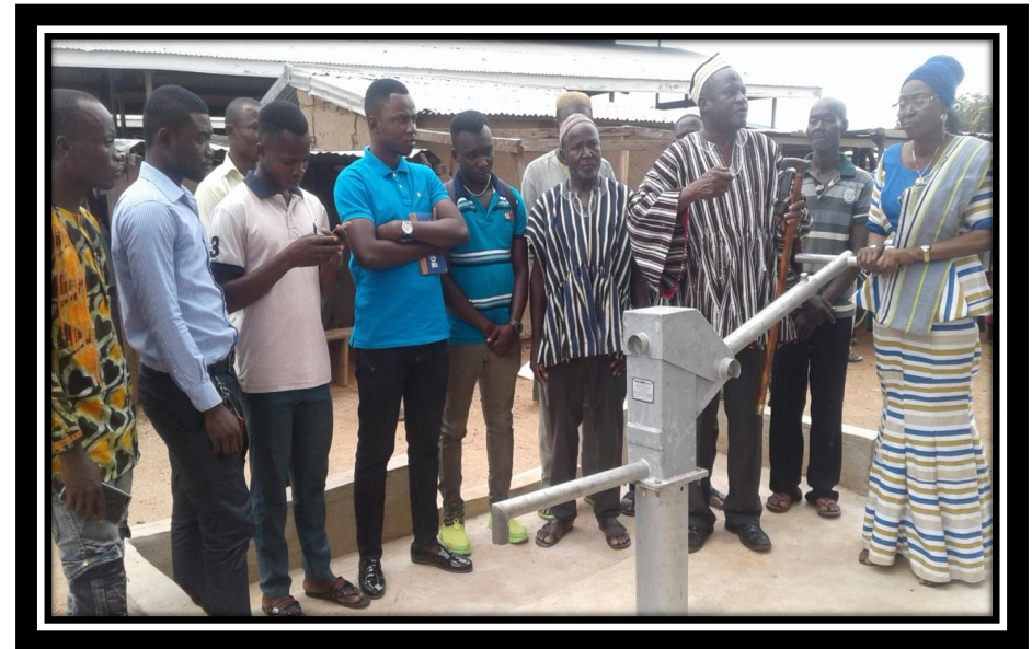
10No. Boreholes constructed
