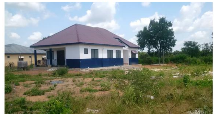
CONSTRUCTED AND FURNISHED 1NO. BUNGALOW FOR DISTRICT POLICE COMANDER
