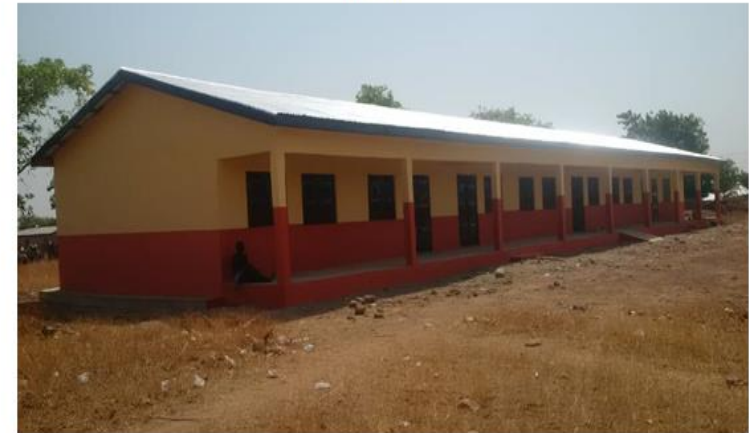
CONSTRUCTED 1NO. 3-UNITS CLASSROOM BLOCK WITH ANCILARY FACILITIES AT KAGBAL
